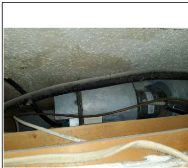
Interior portion of a/c located above the bathroom ceiling
