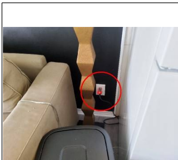
Outlet to the left of the refrigerator is wired reverse polarity
