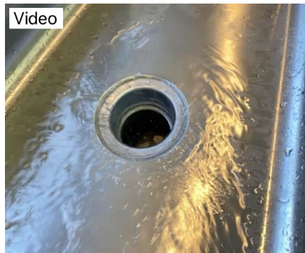
Disposal was operational at time of inspection
