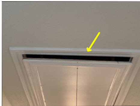
Attic ladder door does not fully close to seal gaps and prevent conditioned air loss.
