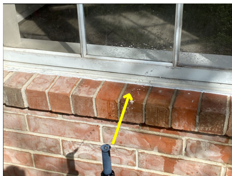
Zone 3 spray heads need adjustment for proper yard cover and reduced over-spray on the house, fence, and paved areas.
