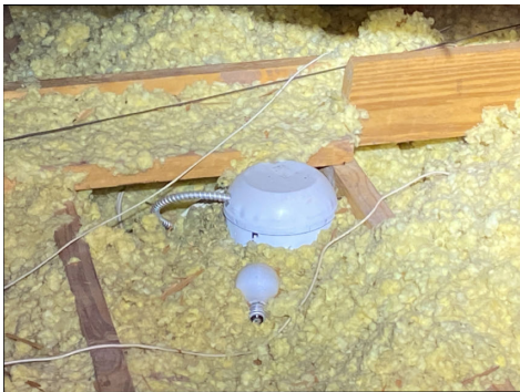
It is a fire hazard for insulation to be within 3" and wood to be within 1" of recessed lights.
