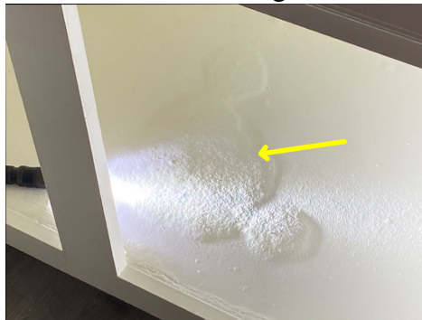
Water damage observed master bathroom West sink
