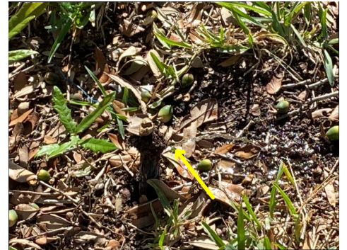
Zone 1 spray heads are clogged and / or grass has grown over head, blocking / preventing proper operation.
