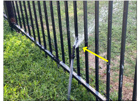
Damaged water line, water gusher in the yard; Station 3
