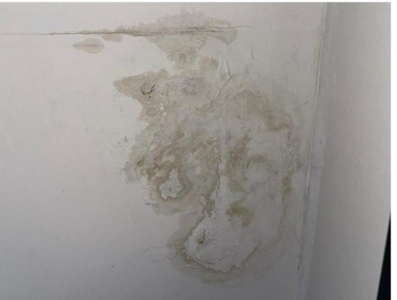
Deficiency: Discoloration from water is present on the doorjamb between the front entry and the living room. This indicates that the roof above this area may allow water to penetrate into the structure. A roofing contractor should evaluate the roof above this area and make any necessary repairs.
