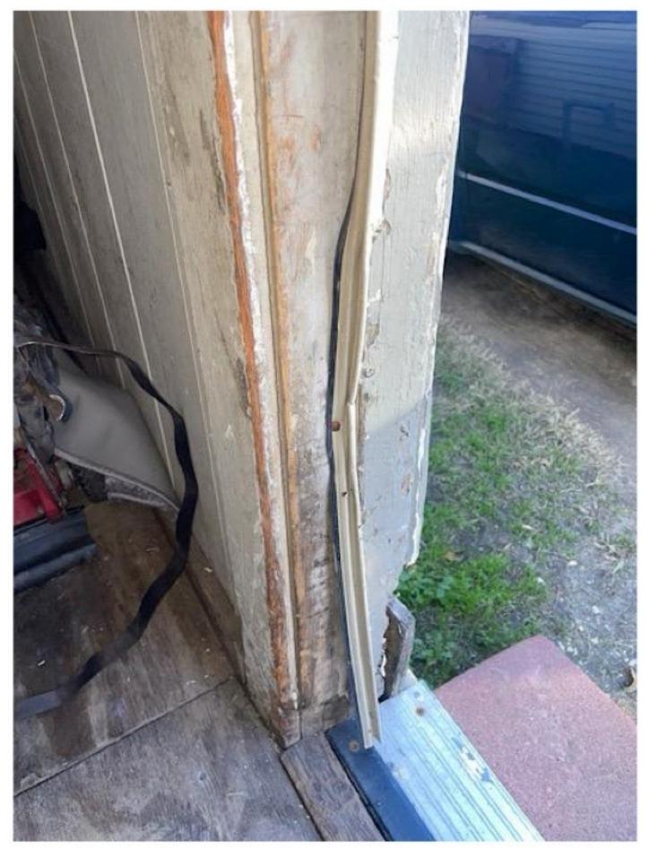
Deficiency: The exterior door on the back of the home is damaged and rusted.
