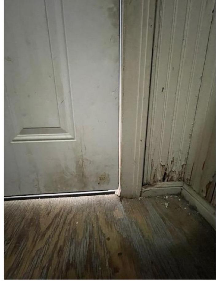
Deficiency: Weather stripping is damaged at all exterior doors.
