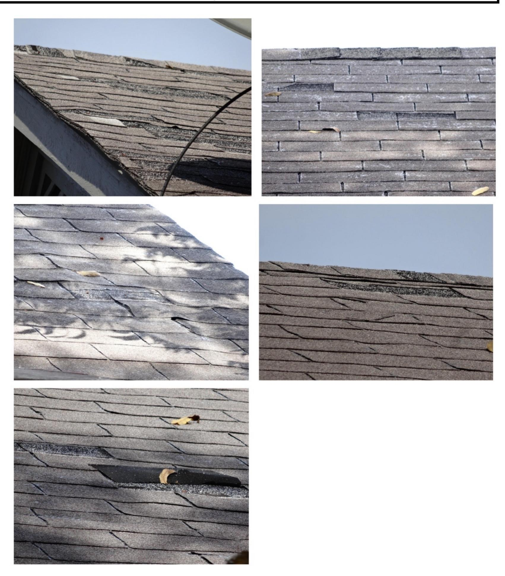
Deficiency: Composition shingles are installed over wood shingles. Wood shingles should be removed and roof decking should be installed.
