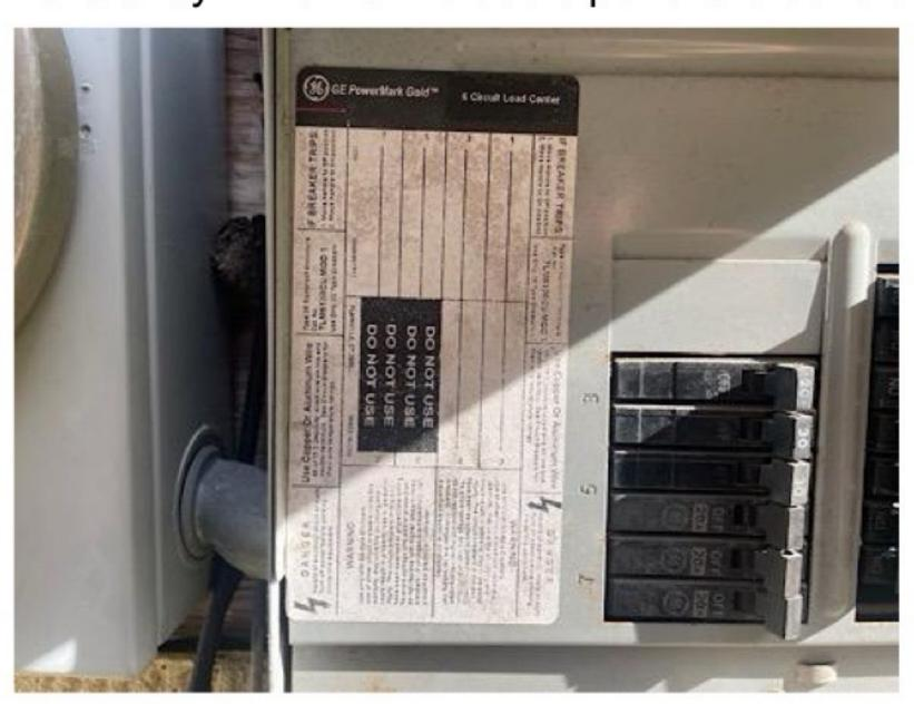
Deficiency: The open space in the main electric panel should be properly covered.
