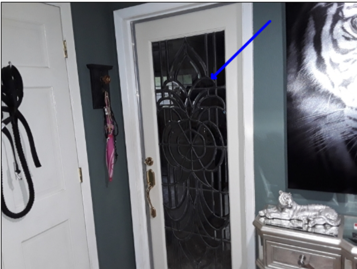
-The garage entry to home is not the proper fire rated door.
