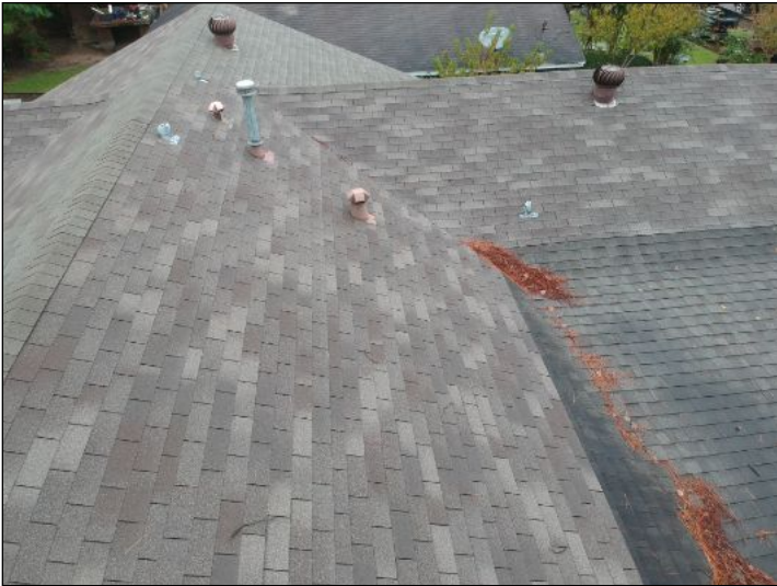
Overview of roof
