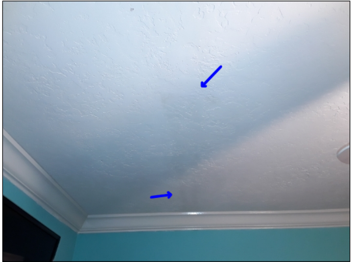
-Checked water stain with a moisture meter and found it to be at a normal level. Unable to determine condition of the underlying materials. Mainly at - middle bedroom
