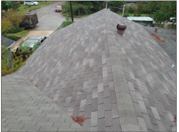
Overview of roof
