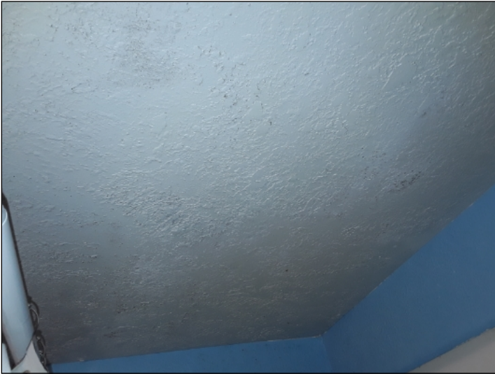
-Mold like stains are present, recommend remediation or cleanup as needed. Unable to determine condition of the underlying materials. Mainly at - above shower at hall bath
