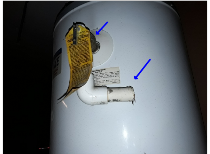
-There is no drain line for the water heater T&P (Pop-Off) valve.
