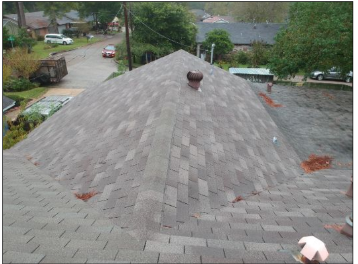
Overview of roof
