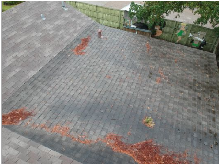
Overview of roof
