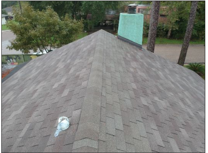
Overview of roof
