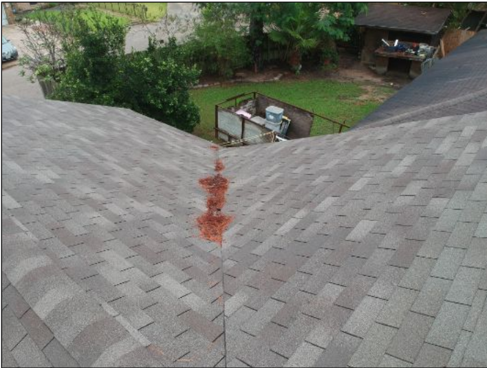
Overview of roof
