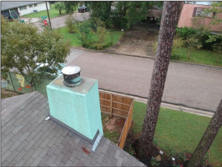
Overview of chimney
