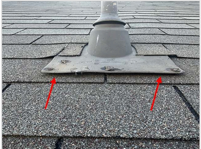
Raised flashing (right)
