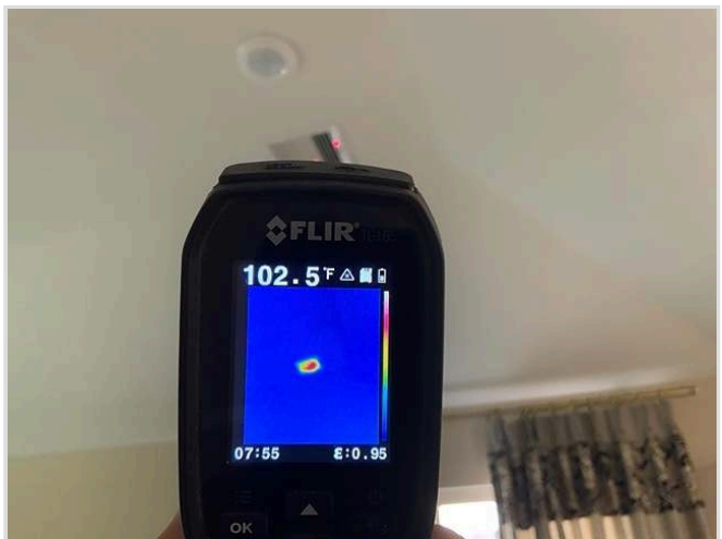
Thermal showing +100 degrees at supply register (dining room)
