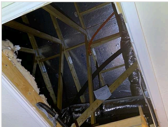
Installed radiant barrier
