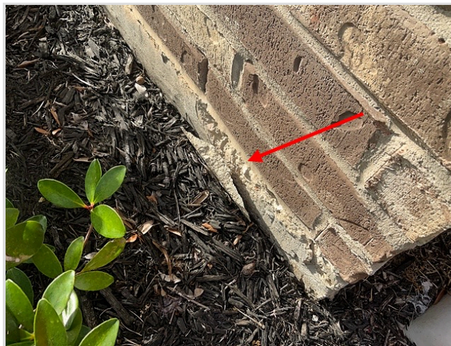
Spalling (front)
