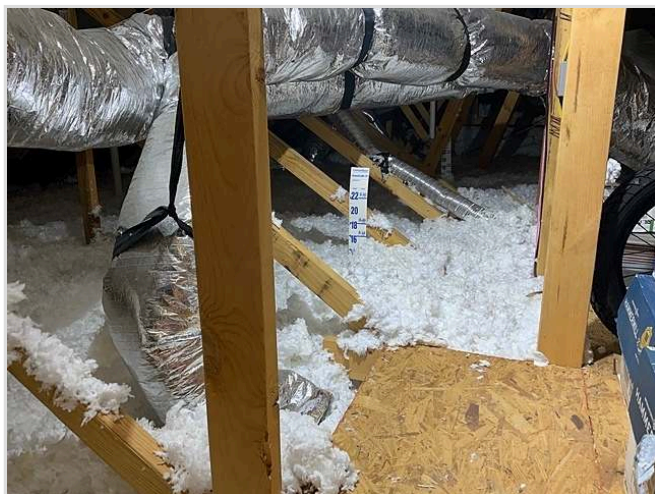
Insulation depth (14-16 inches)
