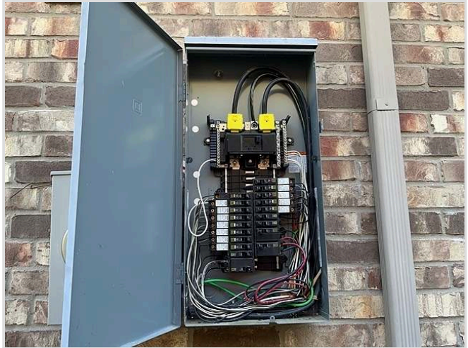
Panel cover removed for inspection
