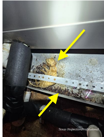
Rodent droppings and dead animal in attic - Recommended professional to deal with the removal and decontamination
