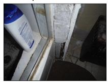
Front wall near baseboard has previous signs of fire. Recommend further investigation and repair as needed.
