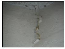
K Hallway shower area is not well sealed. Recommend having bathroom areas repaired as needed and all areas fully sealed.
