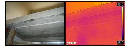
Noted multiple area of damaged ceiling, some with water staining that need further investigation. Repair or replace as needed in all areas affected.
