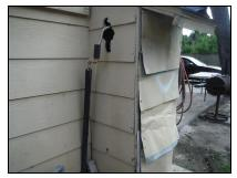
Noted the water heater flue is improperly installed and located to close to home structure and the overhang above. Recommend having licensed plumber further evaluate and repair as needed.
