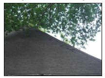
The shingles are worn with significant granular loss in various areas, some shingles are missing at rear. A roofer should perform a maintenance check on the covering for needed repairs, patching or replacement of worn shingles.
