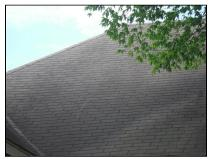
In the shingles are lifting in various areas throughout the roof. These can become further damaged during storms or high winds. Recommend qualified roofer to reseat and apply roofing adhesive to lifted areas of shingles.
