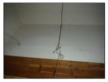
Replace missing cover plates on various outlets and switches. Prevent access to live components that can cause injury or electrocution.
