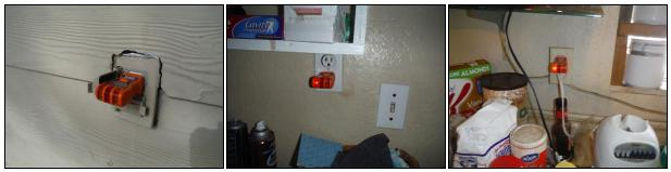
X There was an ungrounded circuit observed in most if not all rooms. The cause should be diagnosed and repaired by a licensed electrician.
