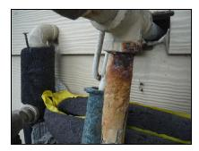
Supply pipes in in the crawlspace/Exterior must be properly insulated. Current condition will not protect piping during hard freeze periods
