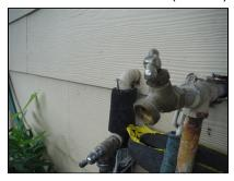
Noted areas of rust at connection points of galvanized piping at exterior and crawlspace. Noted no active leaks at time of inspection.
