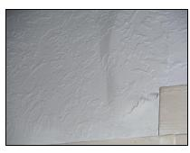
The foundation skirting is cracked in several areas. Mortar repair is recommended to reduce water runoff entry into the crawlspace.
