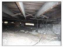
Noted no floor insulation as required by today's standards. Recommend adding insulation at crawlspace floor joist.
