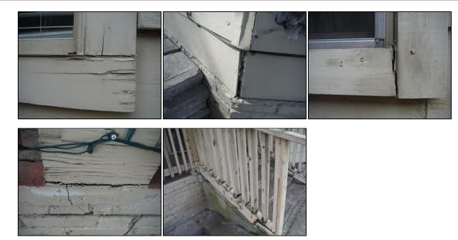
It is recommended that all protrusions through the exterior siding and fixtures mounted on the exterior be sealed in order to prevent moisture incursion. Using a quality exterior caulk type sealant around pipes, wires, light fixtures etc. can prevent moisture related failure of electrical components and siding materials.
