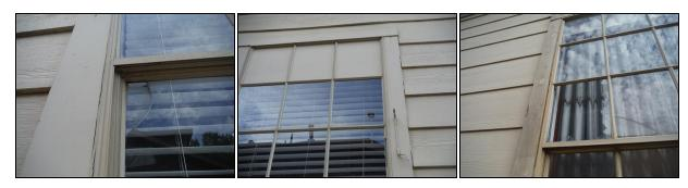
This house is equipped with burglar bars that are not operable. Burglar bars must be removable without the requirement of special tools, special keys or special knowledge for proper egress in the event of a fire. As a general safety rule, we recommend complete removal/replacement of these systems.
