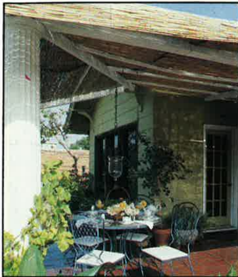
Above: Antique columns, a supporting frame, and a bamboo-reed overhang make up this original structure designed by co-owners Bill Boswell and Byron Franklin.
