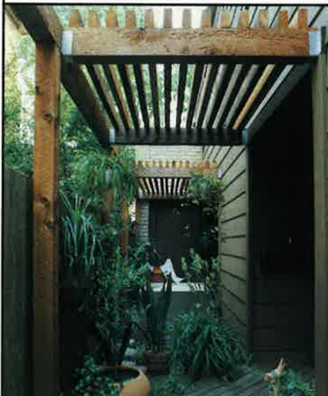
Above: Shading a west-facing exposure, this structure was designed by architect Tom Stovall for his own townhouse. The 2x4s are positioned perpendicular to the path of the sun, allowing dense shade by mid-afternoon. But the openness of the design allows for cooling air movement.
