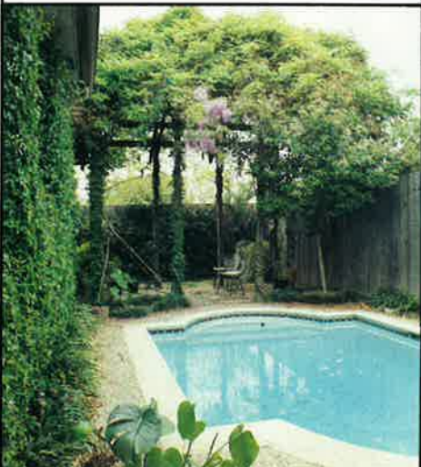
Above: Shading a west-facing exposure, this structure was designed by architect Tom Stovall for his own townhouse. The 2x4s are positioned perpendicular to the path of the sun, allowing dense shade by mid-afternoon. But the openness of the design allows for cooling air movement.
