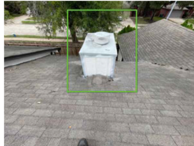
Chimney structure at roof
