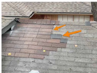
At patch near front roof
