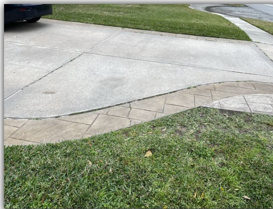
Cracking was found at sections of the driveway.
