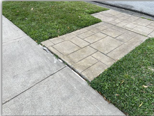
Cracking was found at sections of the driveway.
