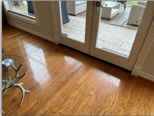
The wood floors are showing signs of wear and tear (ding's, scratches, etc.).
