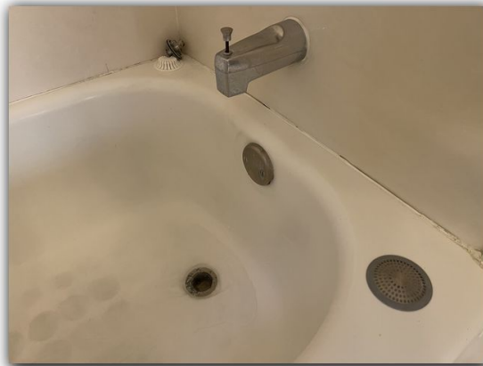
Damaged and missing grout/caulking was noted in the left guest bathroom shower/bathtub enclosure.
