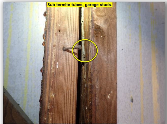
Sub termite tubes, garage studs.
