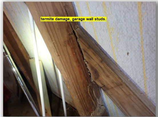
Sub termite tubes, garage studs.
