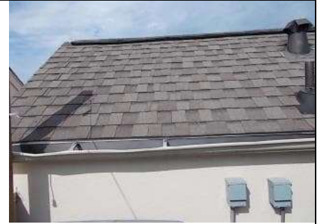
Roof Viewed From Deck
