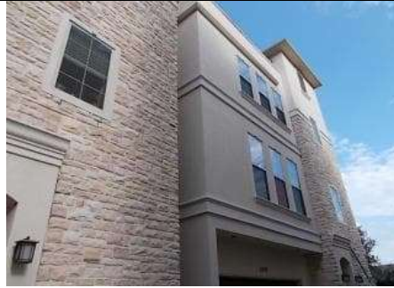
Roof Viewed From Ground
