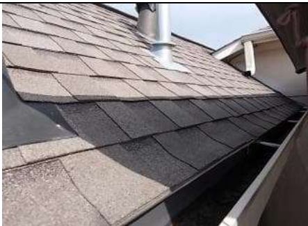
Roof Viewed From Deck
