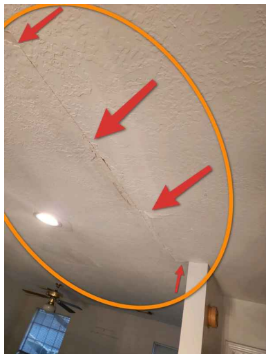
2nd Floor media room
