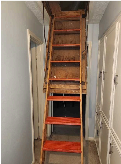
Missing insulation
