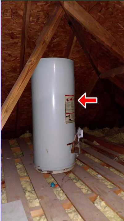
C. Item 7(Picture) upoer attic
