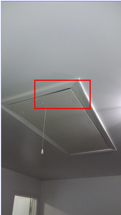
D. Item 1(Picture) garage
