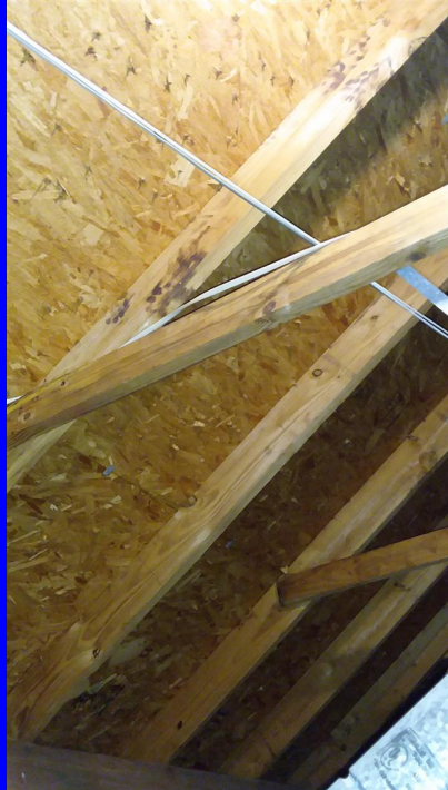
stick built roof structure
