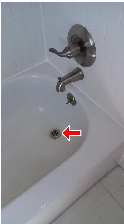
B. Item 2(Picture) hall bath
