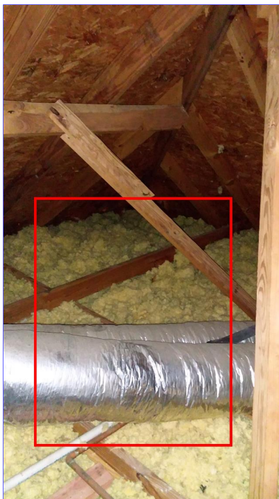
D. Item 7(Picture) upper attic
