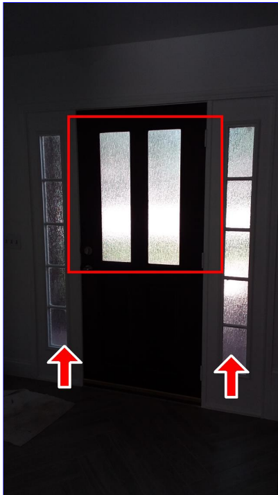
H. Item 3(Picture) entry
