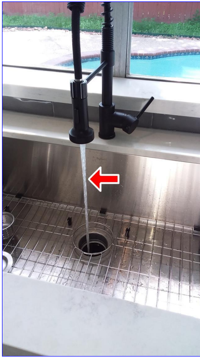
A. Item 4(Picture) kitchen sink
