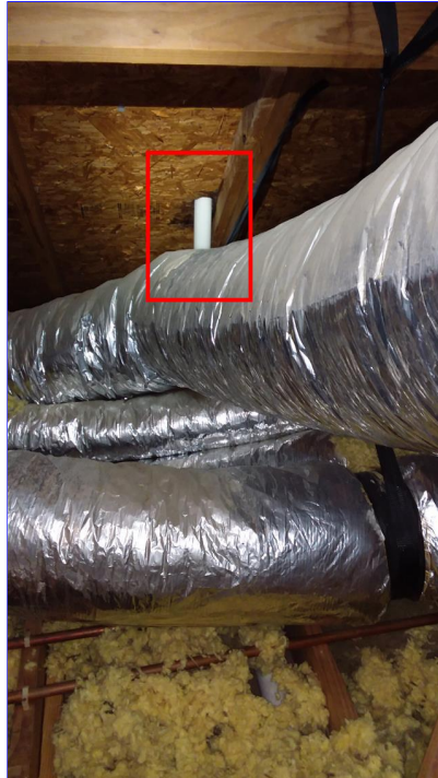
D. Item 10(Picture) rear right
