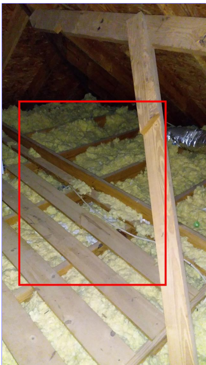
D. Item 6(Picture) upper attic
