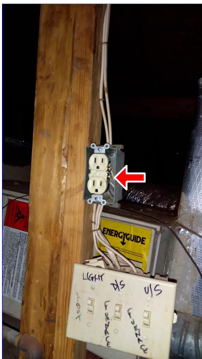
B. Item 8(Picture) upper attic
