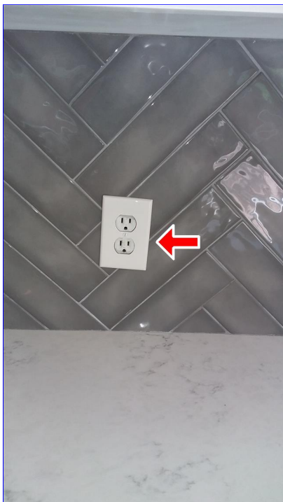
B. Item 24(Picture) multiple outlets
