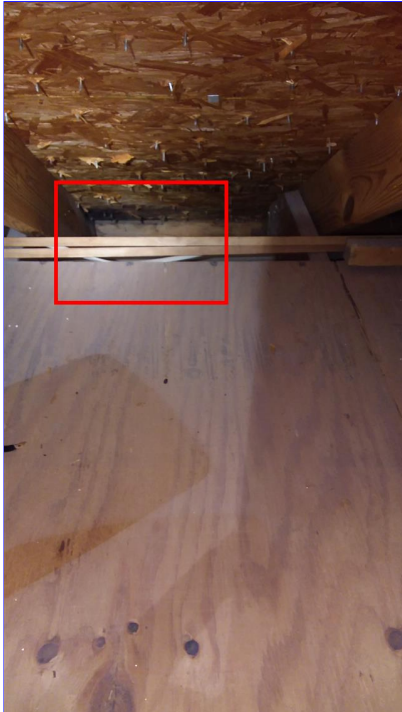
D. Item 9(Picture) garage attic right
