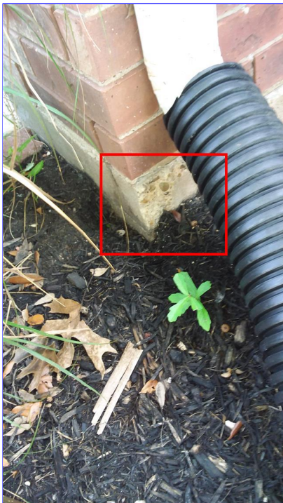
A. Item 1(Picture) garage right
