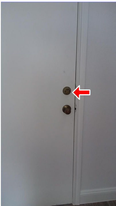
G. Item 5(Picture) garage
