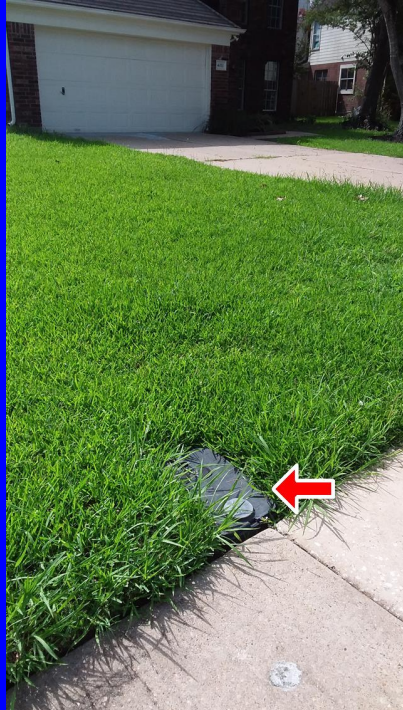
water meter front left
