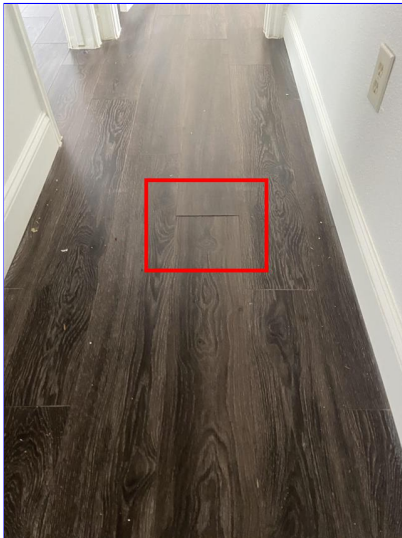
F. Item 1(Picture) hallway upstairs
