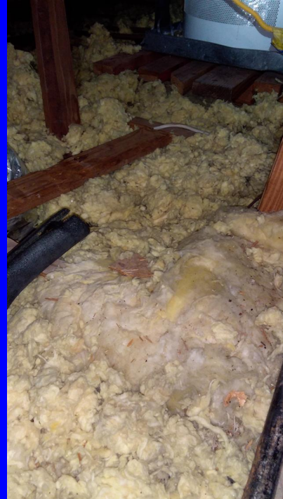
blown insulation 8 inches
