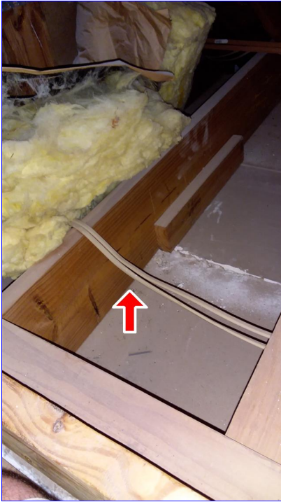
B. Item 9(Picture) garage attic
