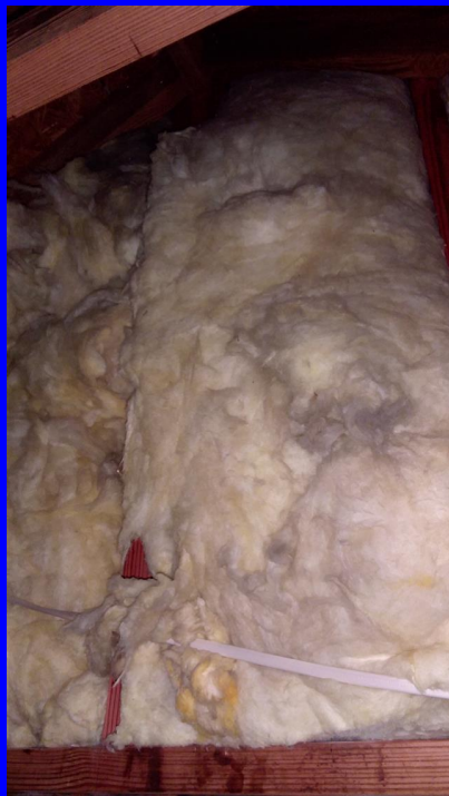
vertical insulation 12 inches
