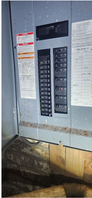
First Sub-Panel Amperage: 200 Amp
