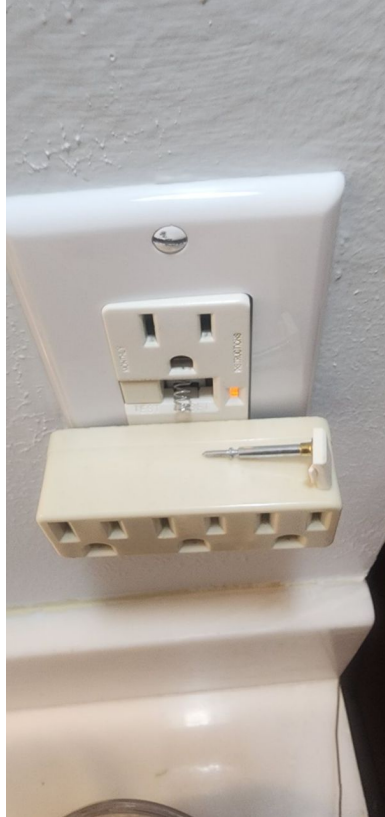
2nd Floor West Bathroom
