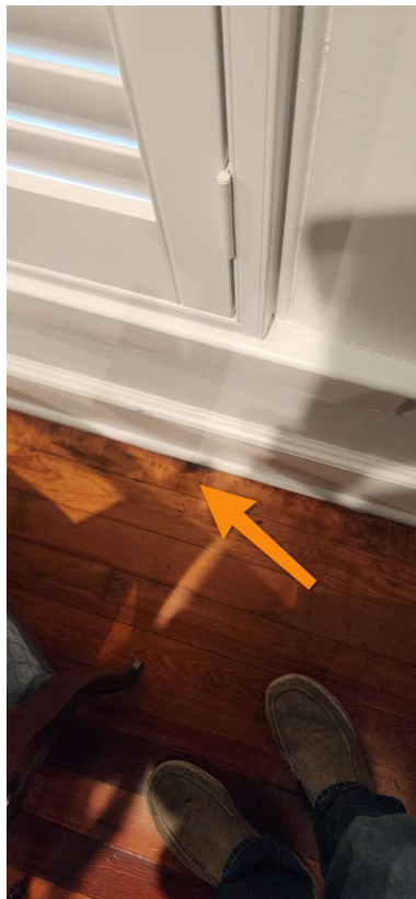
2nd Floor West Bedroom Southwest
