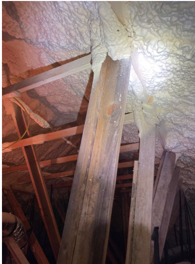
Structural Systems Roof Structure and Attic
