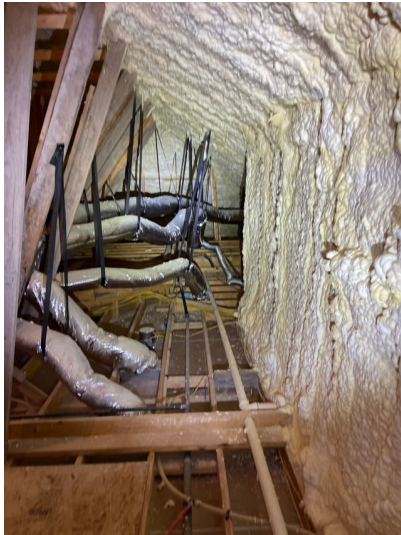
Structural Systems Roof Structure and Attic
