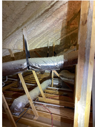
Structural Systems Roof Structure and Attic
