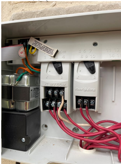
Controller was a RainBird ESP Me timer with 7 stations available and expandable, 6 were currently controlling zones in the yard.
