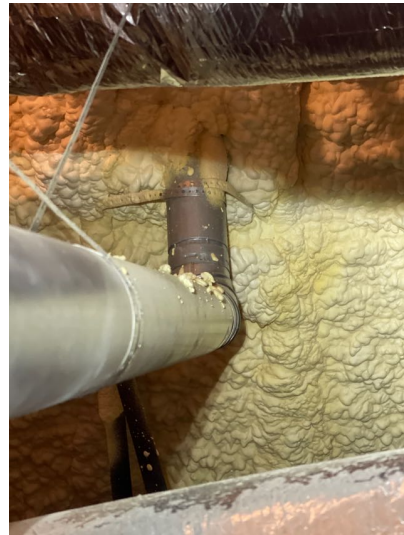
Structural Systems Roof Structure and Attic
