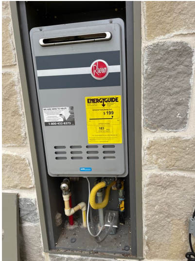
Water heater was gas powered and appeared to be manufactured by Rheem.
