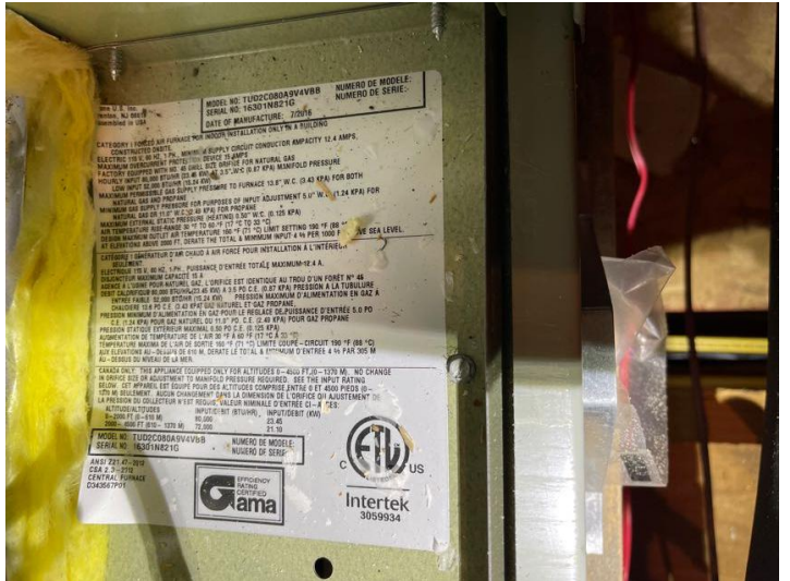
A forced air type, natural gas fired, standard efficiency furnace located in the attic was manufactured by Trane in 2016. Furnace serviced the home with 80k btu's. Furnace was operated, covers were remove and interiors observed.
