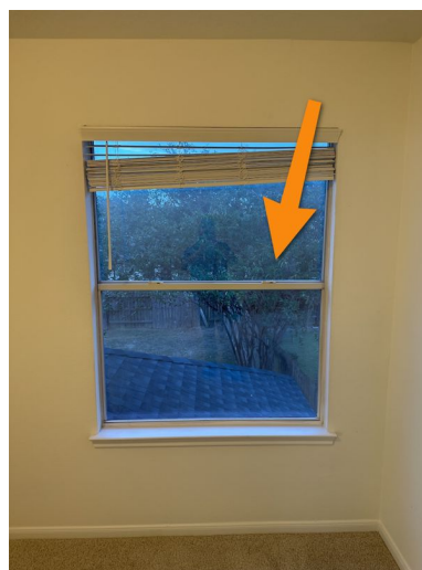
Back 2nd Floor Bedroom
