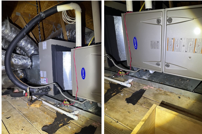
Interior - photo(s) of 2nd cooling system: None 1st unit - measured temperature differential: Low (0°F to 15°F)
