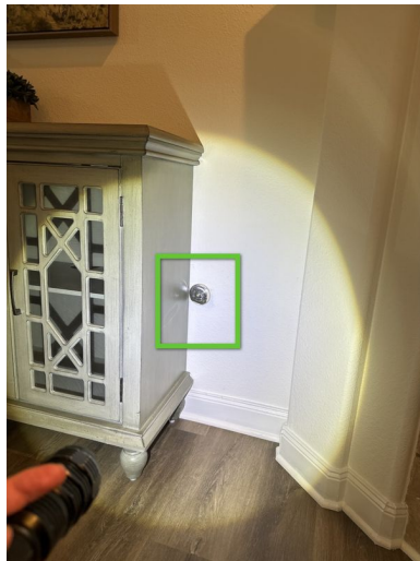
Type of fireplace (w/ photos): Gas Log
