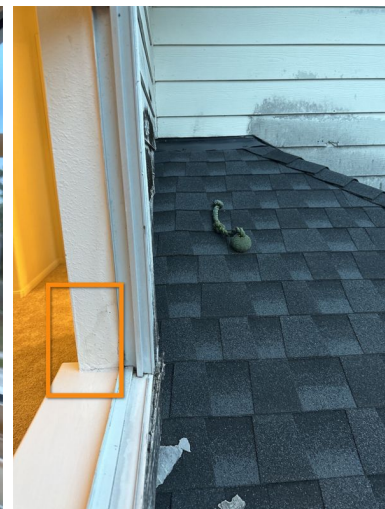
2nd Floor Back Bedroom
