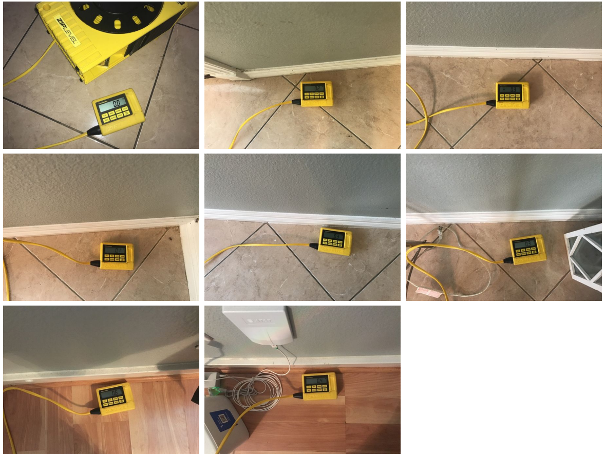
Foundation Inspected with Digital Level:
