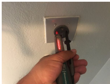
General Photos of Grounding System(s):
