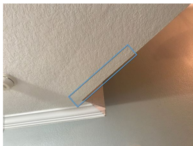
1st Floor Staircase
