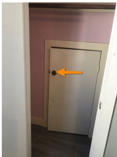
2nd Floor Rear Attic Access
