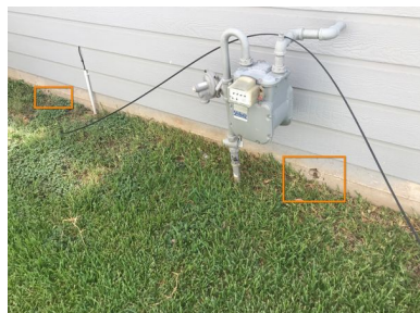
Left Exterior Utility Room
