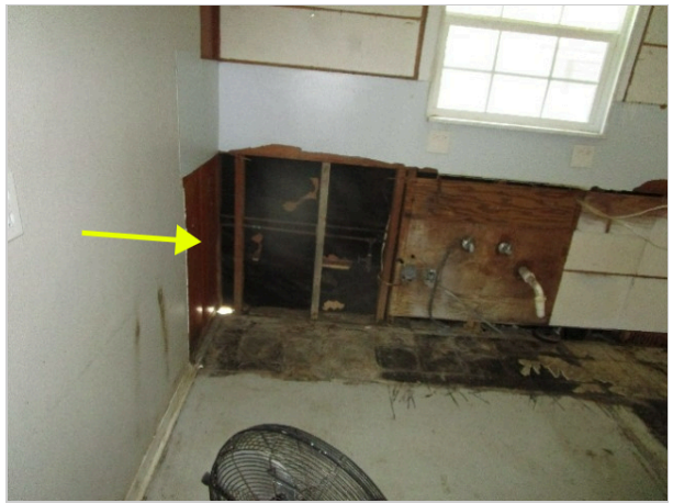
kitchen partially gutted
