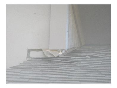
Flashing at the left side of the home should be flush to the roof decking to prevent water penetration into the home.
