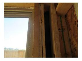
> Headers should be filled with liquid nails to prevent movement.
