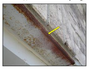
Caulking/paint missing and/or deficient around vertical trim boards may allow wind-driven rain entry.
