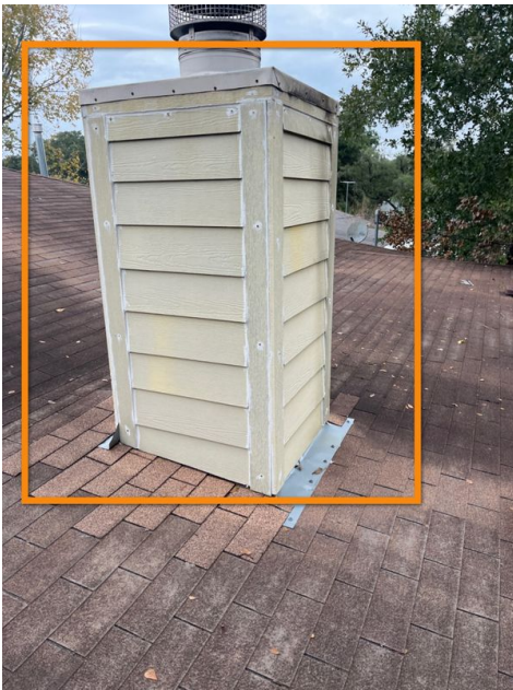
Roof Line Areas
