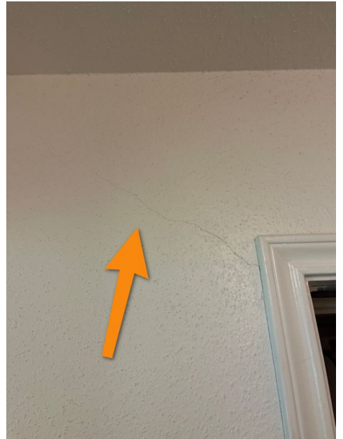
Laundry Room garage door
