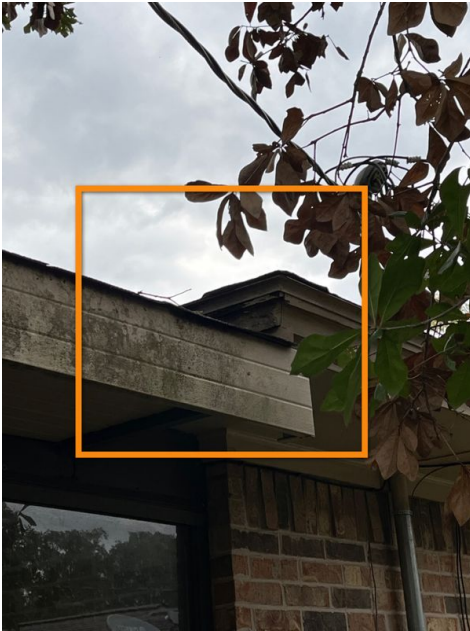
Roof Line Areas
