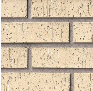
BRICK WALL AND PLANTERS
