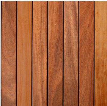
REAR PORCH CEILING
