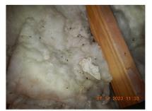
Z Evidence of rodent activity observed at the attic. Further evaluation by a licensed pest control company is recommended.
