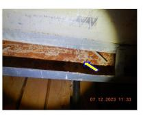
☑ Rust observed at the A/C auxiliary drain pan. Continue to monitor.
