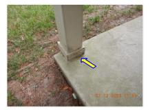
$\square$  Siding at the patio is in direct contact with the flatwork. Water that accumulates at this location can cause the siding to rot/deteriorate.
