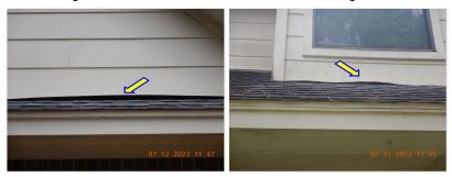
$\square$  Some of the flashing has come up from the roof surface and should be re-secured. ROOF JACKS:
