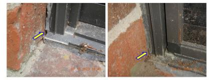
☑ Caulking around exterior windows deteriorating.
