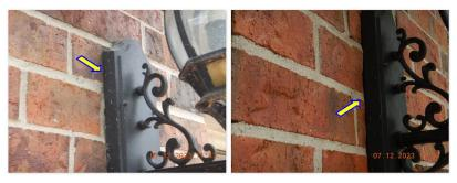
I Caulking/sealant is missing around the exterior light fixtures where missing/deteriorated.
