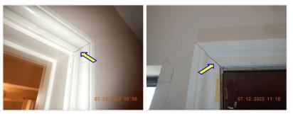
$\ensuremath{\boxdot}$  Door miter joints are separated at some locations.
