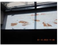
$\ensuremath{\boxtimes}$  Signs of moisture staining on the window sills were present on the windows at the time of the inspection.
