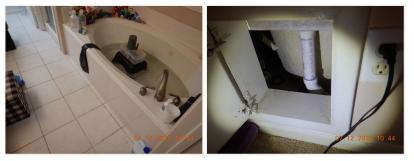
$\square$  The hydro-massage therapy tub at the master bathroom is not installed with an easily accessible inspection panel. The circulation lines and pump/motor could not be visually inspected at the time of inspection. A panel is present but the equipment is not accessible.
