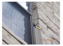
$\blacksquare$  Mortar is missing at some areas of the stone/brick work.
