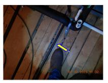
Gas pipes and/or wires and/or water lines are crossing directly over the top of the attic service walkway.
