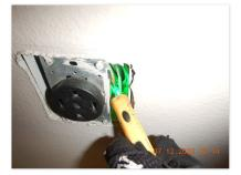
☑ The 220V dryer outlet did not have electrical current at the time of inspection.
