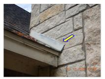
☑ Kickout flashing missing and or inadequate at some locations.
