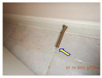
Door stop spring rubber covers are missing at some locations.Door missing at the following locations: Laundry room.
