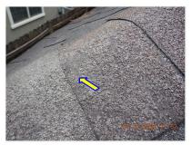
☑ Excessive aggregate loss observed at ridge cap shingles was noted. FLASHINGS:
