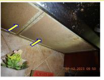
☑ Filter for range hood is dirty or blocked with debris.
