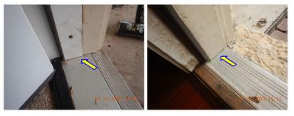
☑ Caulking around the door missing or deteriorated. Some Examples: Back patio, Front entry. Garage Doors Deficiencies:
