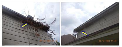
$\square$  Ivy or vines observed attached to the exterior dwelling walls at the following locations: Right side, Back side. Ivy or vines attached to the dwelling can deface or deteriorate the exterior veneer, trap moisture against the exterior wall of the dwelling and create conducive conditions for wood destroying insects.
