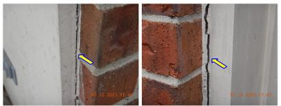
☑ Vertical trim caulking missing or deteriorated. LINTELS:
