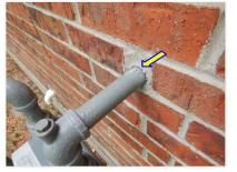
$\square$  The gas lines are not properly sleeved or wrapped with PVC plumbing tape where passing through the exterior veneer at the following locations: Left exterior hose bib.
