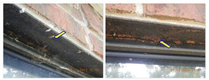
$\ensuremath{\boxtimes}$  Metal lintels are rusting above the doors and windows. FLASHING
