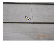
☑ Cement board siding damaged at corner fasteners. CAULKING:
