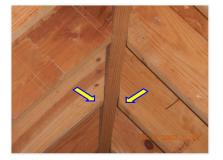
$\square$  Purlins at the attic are undersized. The purlins should be the same size as the roof rafters.
