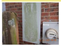
$\blacksquare$  The new NEC changes state that the emergency electric shut off should be labeled with a non-removable plaque.
