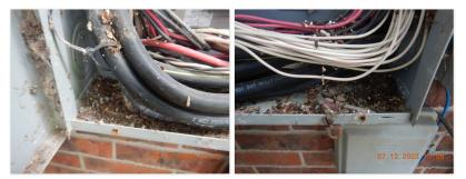
$\ensuremath{\boxtimes}$  Debris observed at the interior of the service equipment disconnecting means panel board enclosure.
