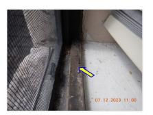
$\square$  Window drainage ports obstructed with dirt and debris. Window drainage ports and other components should be cleaned on a annual basis. Otherwise, drainage ports can be blocked allowing water to back up into the wall area below the windows.
