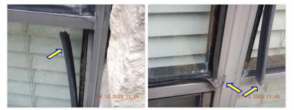
Exterior plastic window strips are damaged at some locations.
