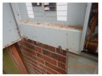
☑ The service equipment disconnecting means panel board dead front cover is rusted. INTERIOR PANEL BOARD:
