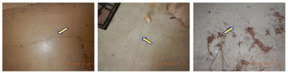
☑ Settlement cracks observed at the flatwork at the following locations: Garage, Front patio, Back patio, Garage.
