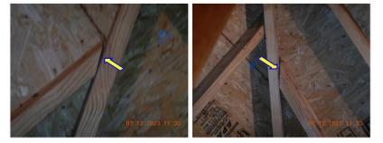
☑ Rafters cuts not flush at the ridge, hip and or valley boards in the attic.
