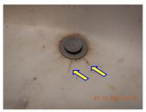
☑ Cracks at the base of the sink observed at the following locations: Master bathroom.
