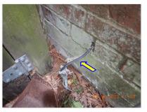
$\ensuremath{\boxtimes}$  The grounding electrode conductor connected to the grounding electrode is not protected from physical damage.
