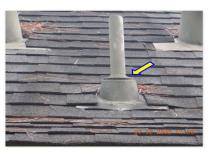
$\ensuremath{\boxtimes}$  The house is old enough to require the boot jacks to be re caulked due to deterioration at the seal or possibly changed.
