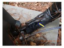
$\square$  Insulation is missing or deteriorated on the A/C suction line at the condensing unit. DRAIN LINES:
