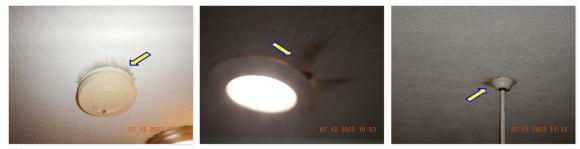
☑ Singe marks were observed around multiple electrical fixtures. *Smoke and Fire Alarms Deficiencies:*
