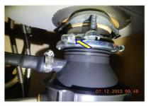
$\square$  The food waste disposal connection clamp is not locked into place at the sink flange. Disposal vibration may cause the unit to leak or detach at the sink connection.
