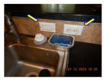
$\square$  Switch and plug are installed at a prohibited location at the kitchen.
