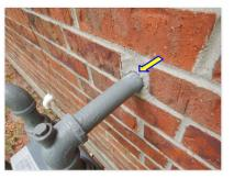
$\square$  The metal gas distribution pipe entering the building should be bonded to the electrical system. The metal gas pipe is not bonded or could not be verified at the time of inspection.
