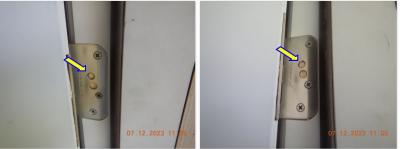
☑ Door hinge fasteners missing at some locations. ☑ Door knobs are loose at some locations.
