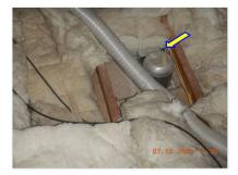
☑ Clear insulation from around the recessed light fixtures at the attic.
