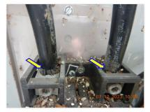
☑ No anti-oxidant solution installed at the aluminum service-entrance conductors termination lugs. *Service-Entrance Equipment Grounding and Bonding:*
