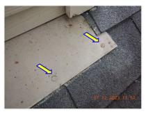
☑ Nail heads are exposed at the flashing and/or composition shingle.
