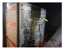
☑ Circuit breaker installed at A/C condensing unit circuit is too large per manufactures specifications. 40 amp installed and 25 amp is required per manufactures specifications.
