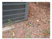
☑ Condensing unit is not installed the proper distance above grade.
