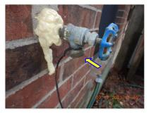
$\ensuremath{\boxtimes}$  Exterior hose bibs not installed with anti-siphon devices at some locations. SINKS:
