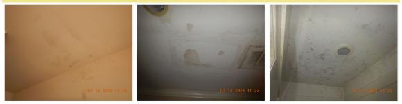
$\boxdot$  Evidence of moisture stains observed. Some Examples: Garage, Master bedroom, Master bathroom, 2nd floor stair landing.
