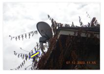
☑ Note: Satellite dish has been installed on the roof. Some satellite dishes and/or mounting brackets have been abandoned. These penetrations should be caulked at the fasteners.
