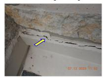
☑ Caulking is deteriorated at some of the roof flashing locations.
