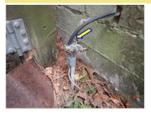
☑ The grounding electrodes should be driven to below top surface of the soil.
