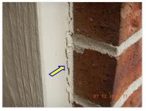
$\blacksquare$  Caulking is deteriorated at the garage door trim.
