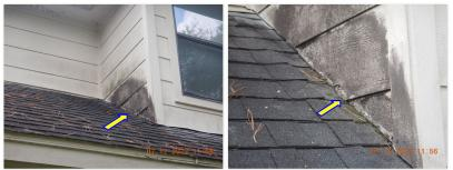
$\blacksquare$  Exterior siding is in contact with the roof. Separation between the siding and roof covering will minimize moisture entrapment and deterioration of the siding.
