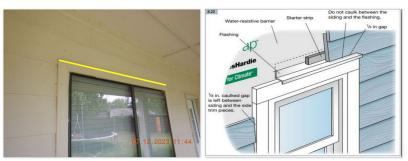
$\boxdot$  The window and/or door and/or other wall penetrations installed through the wood fiber products siding were not properly flashed.
