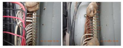
$\square$  Several neutral conductors and grounding conductors are double terminated. The neutral conductors should be installed under separate terminal screws. This is a possible electrocution hazard.
