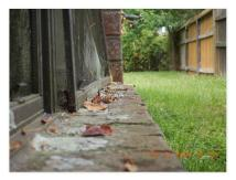
$\square$  Window brick ledges are not properly sloped to shed water. The brick ledge should be installed with a 3/4" slope or at least a 15 degree angle.
