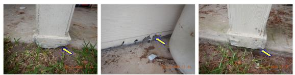
Cement board siding and/or trim damage was noted.Nails in the siding should be pitted and caulked over.
