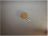
$\square$  Note: Most smoke detector alarm manufactures recommend replacement of the smoke detector after 10 years. Therefore, if the smoke detector(s) is perceived by this inspector to be more than 10 years old it will be recorded as defective and in need of replacement.
