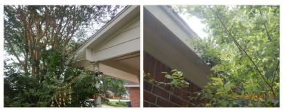
$\boxdot$  The roof has tree limbs coming in close contact with the roof covering. Tree limbs can cause damage to the covering and allow access to the roof for unwanted pest. I recommend trimming back all tree limbs away from roof.
