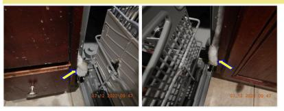
☑ Insulation is sticking out of the sides of the dishwasher compartment.
