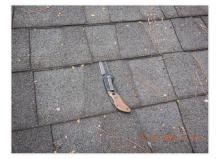
☑ Per the Texas Real Estate Commission Standard of Practice effective February 1, 2009, home inspectors are required to inspect shingle fasteners. To inspect fasteners, the lower tab of the shingle must be lifted at several locations. As is the case in most homes, this inspection was not possible without damaging the shingles. Under the Standards of Practice departure clause this item was not inspected.
