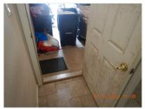
☑ Self closing hinges not properly tensioned at the garage entry door.
