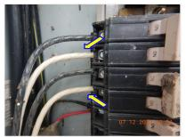
☑ The white wire connected to the 240 volt circuit breakers should be marked with a color (red or black).
