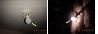
$\boxdot$  Light fixture globes missing at the following locations: 2nd floor front left bedroom closet, Garage, Master bathroom, Attic.
