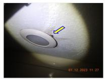
☑ Cracks/damage/repairs in the ceiling drywall observed.
