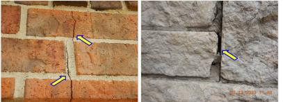
☑ Cracks observed in the brick veneer and/or mortar were noted. <u>SIDING:</u>
