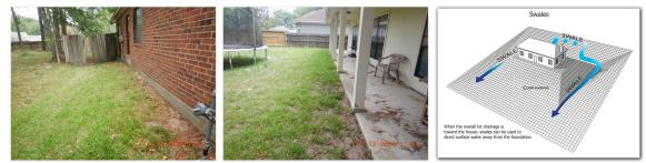
The drainage and grading around this home is inadequate. In order for the drainage to be effective, the landscaping must be configured so that the yard is sloped away from the foundation by at least 6 inches in the first 10 feet and/or adding additional gutters/downspouts to the house is another option to improve drainage and/or in- ground drains should be designed and added to divert rainwater and runoff away from the house as appropriate and/or drainage swale should be improved/installed.
