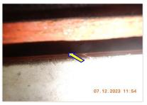
$\blacksquare$  The roofing felt did not extend to the rakes or bottom of the roof deck in all of the areas that were inspected.
