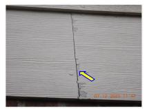
☑ Caulking is needed at all joints and unsealed seams in the siding.
