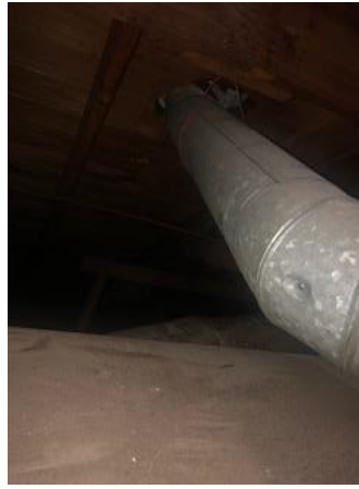
Extend flue pipe through the roof with caps and collar.
