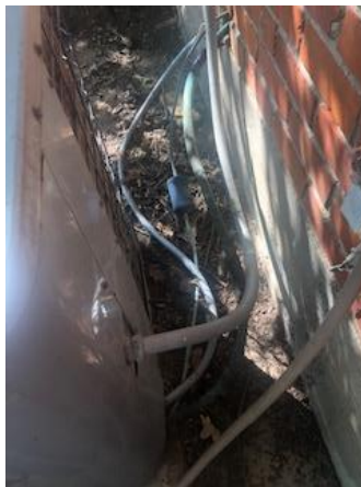
Insulate suction line at condenser.
