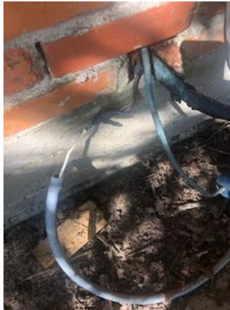
Secure low voltage wire.
