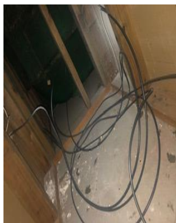
Seal return air chute with duct board.
