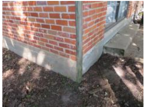
G=Wood To Ground Contact
