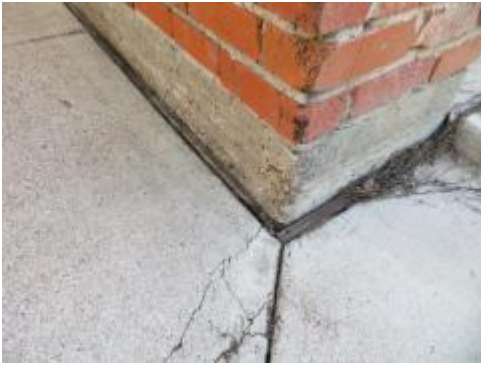
I=Form Boards Left in Place
