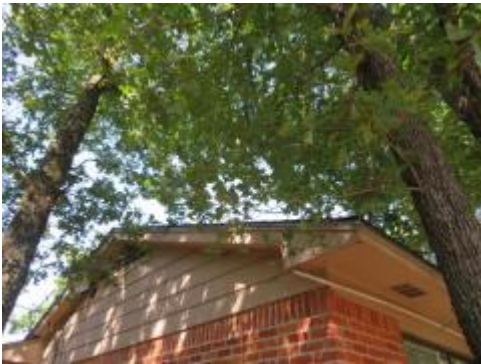
N=Foliage in Contact w/Structure
