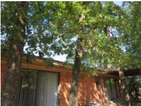
N=Foliage in Contact w/Structure
