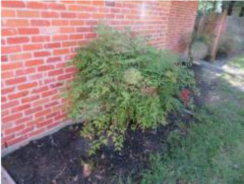
N=Foliage in Contact w/Structure
