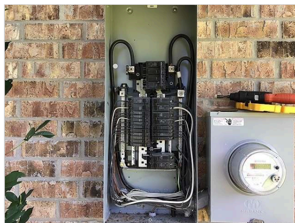
Panel cover removed for inspection
