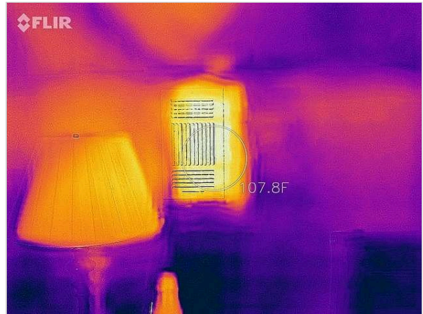
Thermal showing 100+ degrees of temperature output (upstairs guest bedroom)
