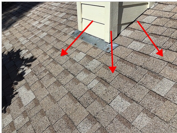
Accelerated granule loss
