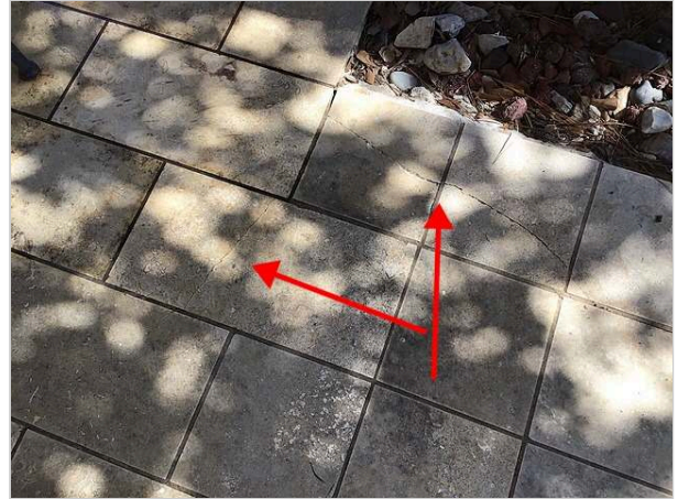
Cracked/damaged tiles
