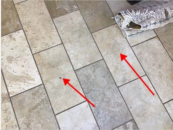
Cracked/damaged tiles
