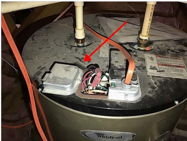
Not installed (cover plate)
