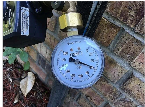
Static water pressure
