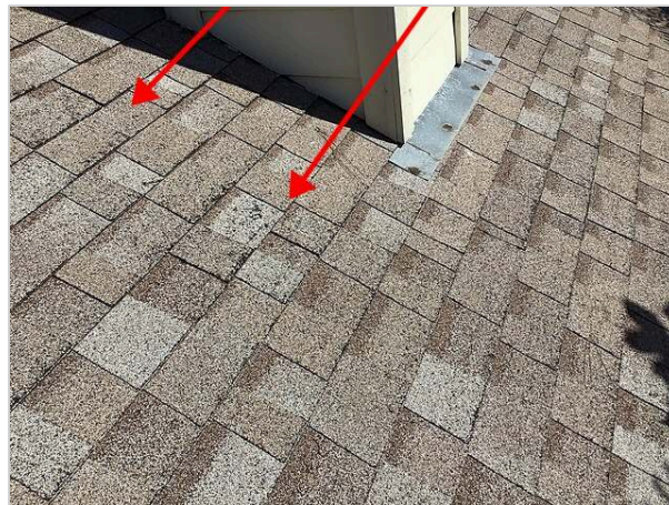
Accelerated granule loss
