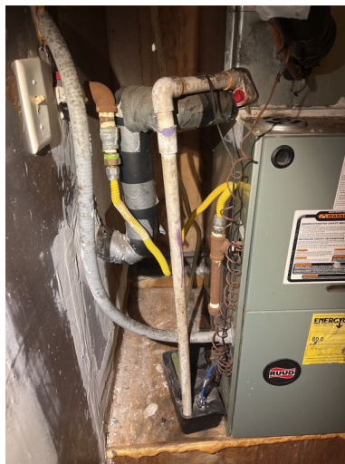
1st unit - measured temperature differential: Operable (15°F to 20°F)
