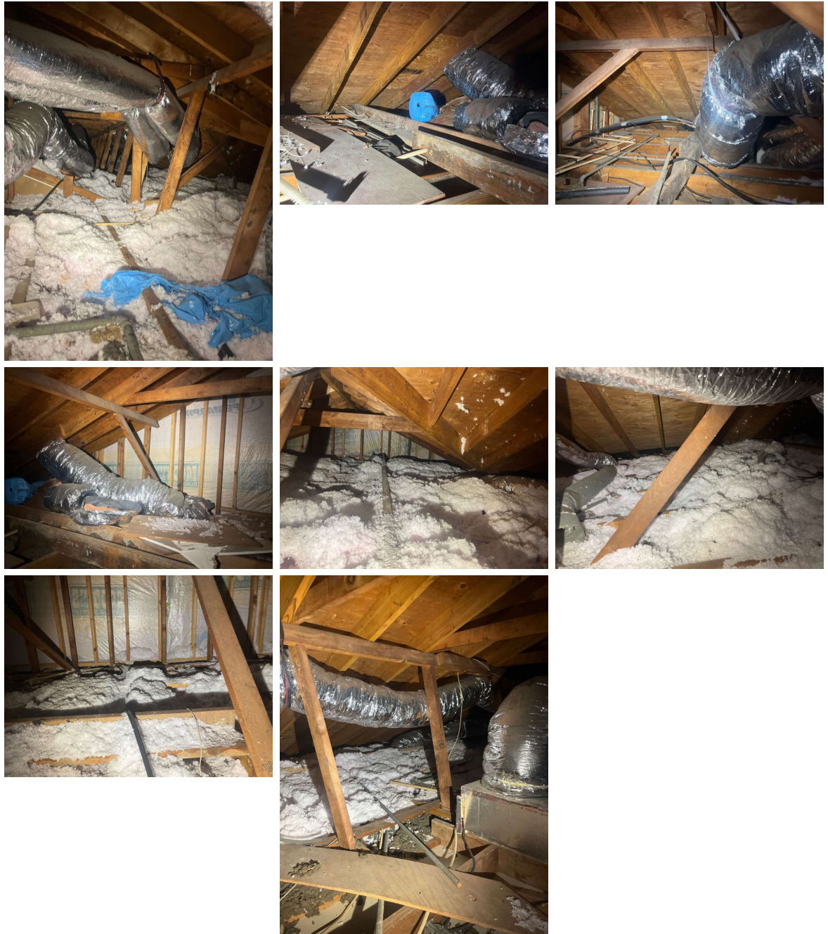
Type of insulation (w/ photos): Blown-In / Loose Fill
