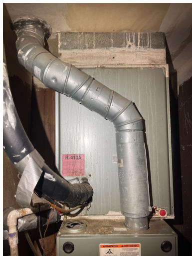
1st unit - measured temperature differential: Operable (15°F to 20°F)
