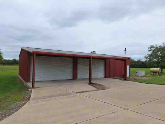
Metal Building with overhang
