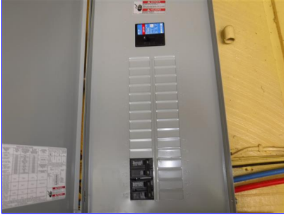
A. Item 1 (Picture) Panel
