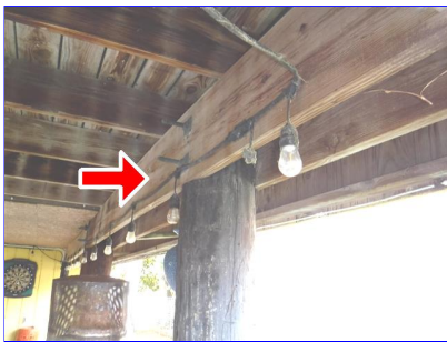
A. Item 1 (Picture) Foundation
