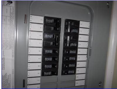
A. Item 4 (Picture) Panel
