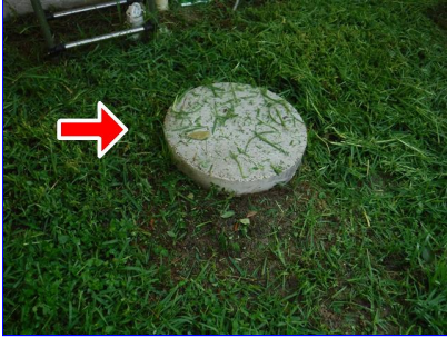
E. Item 1 (Picture) Septic tank rear
