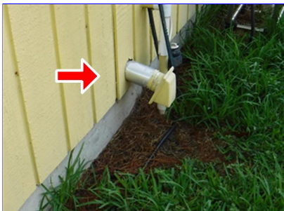
H. Item 1 (Picture) Cut to proper length and seal.
