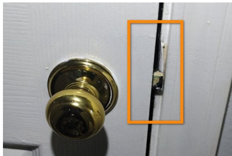
2nd Floor Hall Closet
