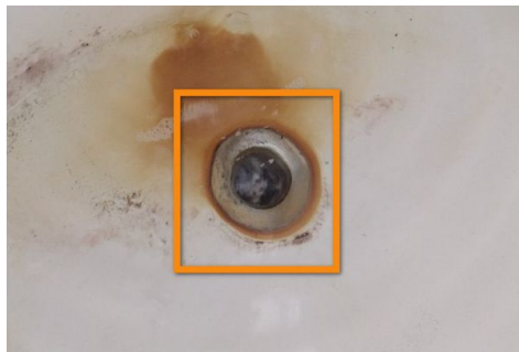
2nd Floor Bathroom
