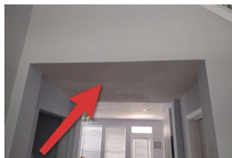
1st Floor Hall
