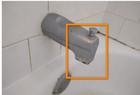
2nd Floor Bathroom
