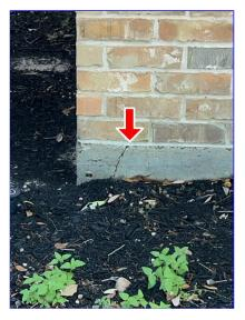
(2) Elevation readings of the slab, with a zip level do not indicate evidence of excessive movement or unlevelness of the slab.
