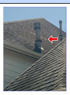
(2) The garage does not have any roof ventilation. At the next roof replacement I recommend adding ventilation to the roof of the garage.
