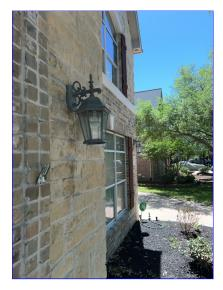
(2) The two Coach lights on the front of the house as well as the Coach light for the garage did not turn on with the switch. Recommend correction.
