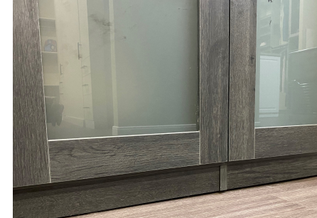
Pulled forward Toe Kick (1) Pulled forward Toe Kick
