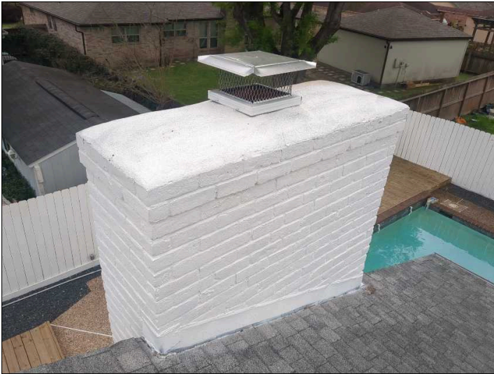
Overview of Chimney.
