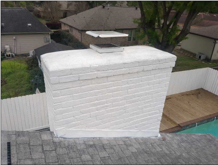
Overview of chimney
