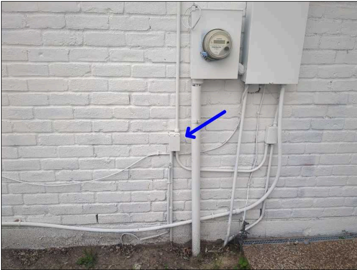
The GFCI (Ground Fault Circuit Interrupter) electrical outlet does not trip when tested. Mainly at - right side exterior
