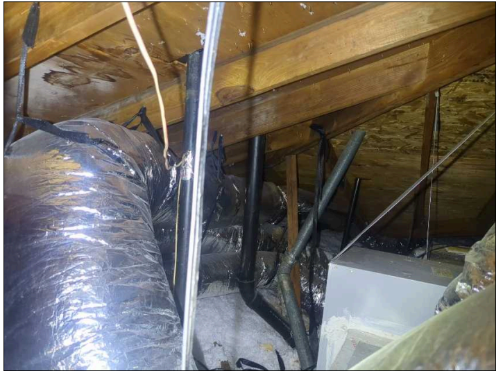
Overview of Attic.
