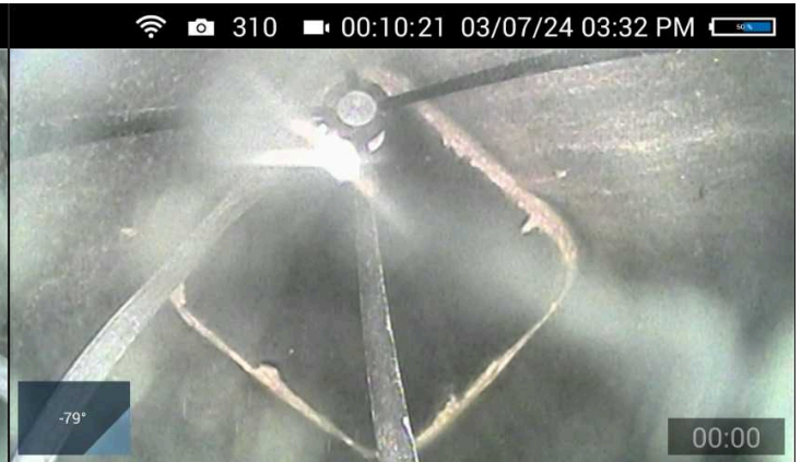
Overview of flue mortar joint
