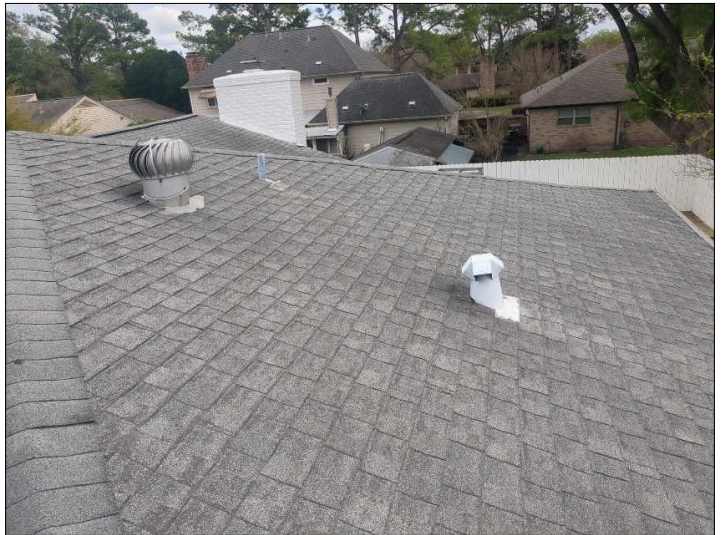
Overview of Roof.
