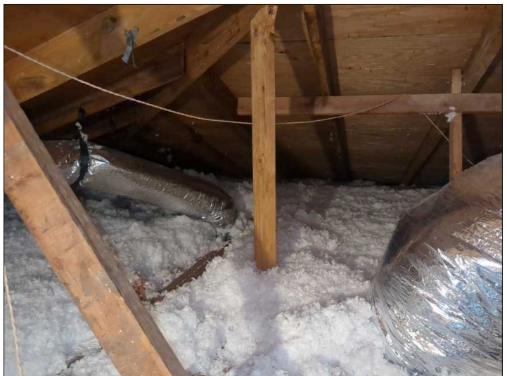
Overview of Attic.
