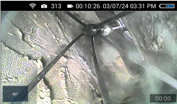
Overview of fireplace smoke shelf
