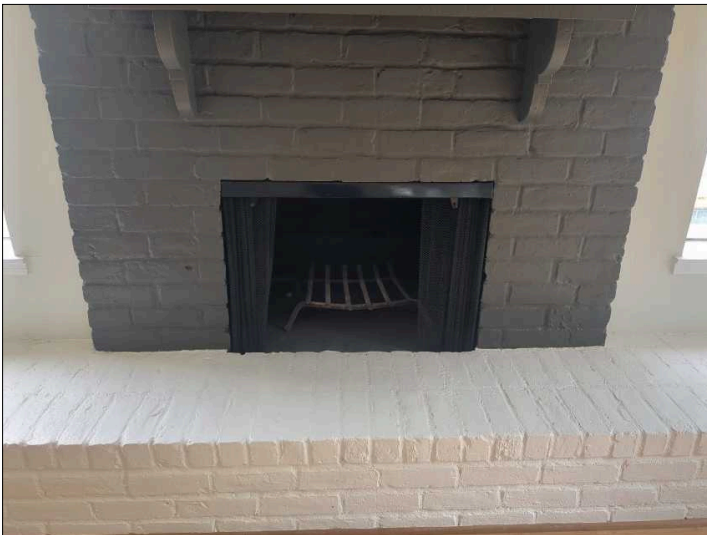
Overview of fireplace
