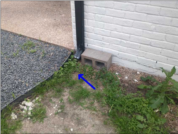
Splash blocks or downspout extensions should be installed to direct water away from foundation.
