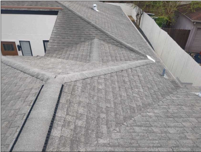
Overview of Roof.
