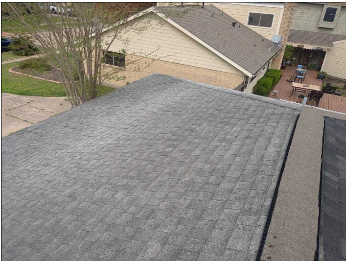
Overview of Roof.
