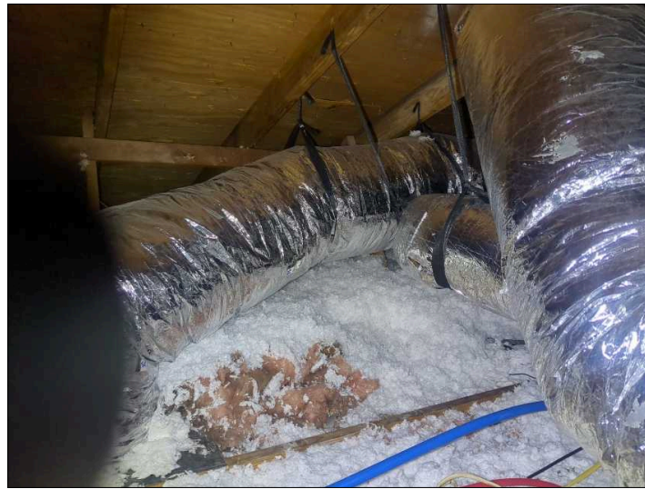
Overview of Attic.
