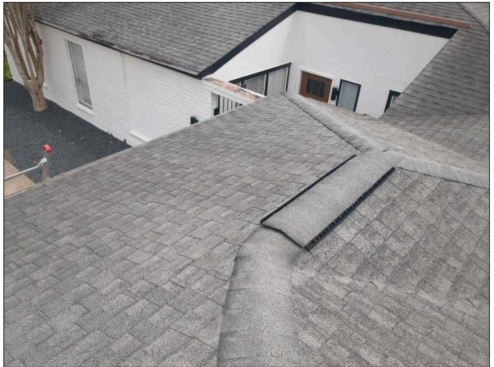
Overview of Roof.
