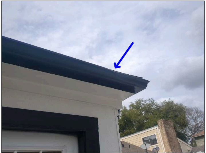
The gutter is bent/damaged. Mainly at - rear left
