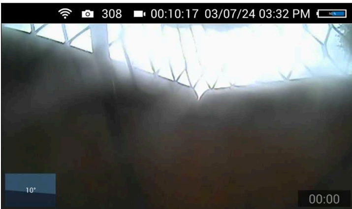
Overview of chimney cap from the inside
