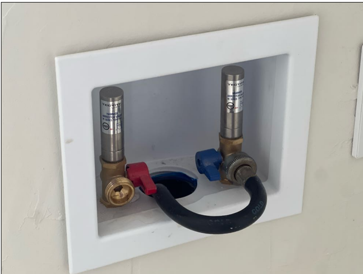
Overview of Laundry Supply and Drain Test.
