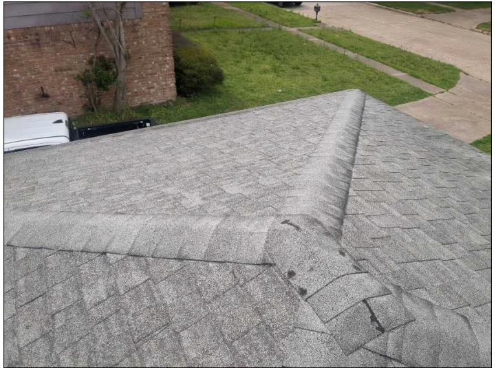
Overview of Roof.
