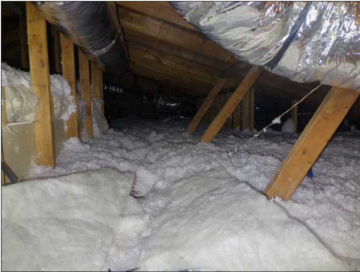
Overview of Attic.
