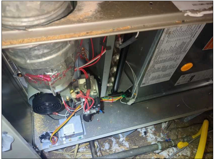
Overview of Furnace burner compartment.
