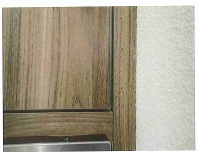
6. Cabinet facings around the oven and microwave oven had been installed with fasteners driven through the face of the facings that were prefinished. This creates an irregular appearance that may not be repairable without replacement of the facings.
