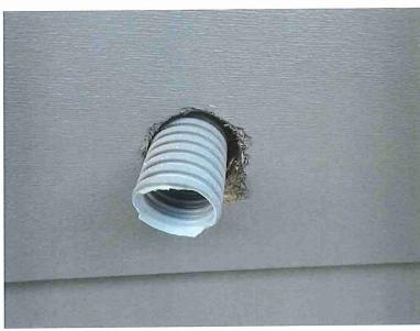
10. Penetrations through the fiber cement siding visible along the east side of the building were apparently made without adequate flashing to the waterresistant barrier behind the siding. The rough edges of the sheathing were visible around some penetrations. This increases the potential for water entry and is generally difficult to properly repair without removal of siding materials.
