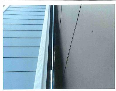
The gutter system at the west side of the building adjacent to the upstairs hall bathroom area was partially crushed, apparently due to a lack of adequate clearance to the adjacent unit. This will reduce its cross-sectional area and increase the potential for it to become clogged. This may increase the need for cleaning. Access to the gutters appears to be only from the roof and will be difficult.
