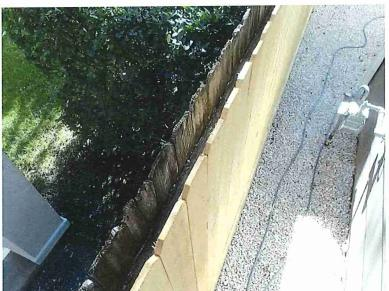
It appears finish nails had been used to secure some siding at the south side of the building. Nails could be observed at other locations. Finish nails are not considered an acceptable fastener for securing siding.
