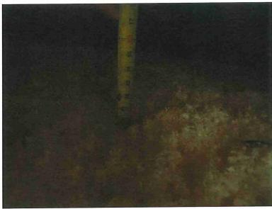
Insulation in the attic space was measured to be less than the R=38 specified on the data tag in the attic and the R=30 specified on the data tag at the panel box. R=38 is the minimum prescriptive depth of insulation acceptable in the Houston area, and there is an apparent need to add insulation at the attic.
