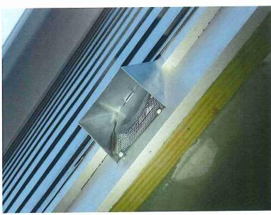
The 1/2 bathroom ventilator fan outlet had a bent damper and did not close tightly against the damper, and the vent flue was not flashed to the water-resistant barrier. Because the hood is not flashed to the water-resistant barrier, this increases the potential for water entry and may result in energy loss since the damper does not close tightly.
