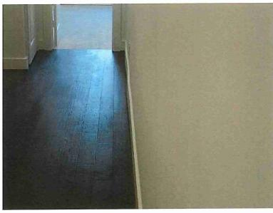
13. The base trim was uneven along the east side of the upstairs hall adjacent to the master bathroom, creating a poor appearance.
