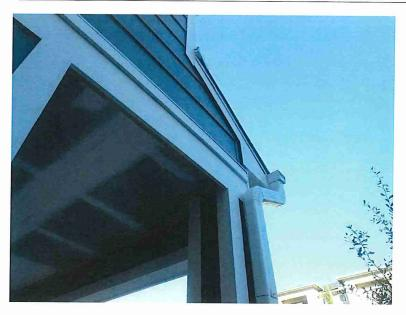
22. Trim at the east side of the carport extended past the upper trim without a flashing detail. This may allow water entry behind the trim components at the corners of the column and front wall.
