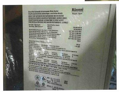
3. Hot water for the building was provided by a single on-demand gas-fired water heater having a maximum input capacity of 199,000 BTU/hr. Determining the adequacy of the water heater was beyond the scope of this inspection and should be designed based upon the maximum flow anticipated and the required temperature rise for an on-demand water heater. The equipment appeared to be of a size typical {...full text in report}
