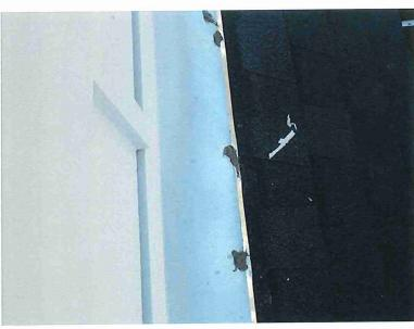
The roof head flashings had fasteners driven exposed in the lower surfaces to hold the flashing down against the roof. If the flashings had been properly constructed, there would have been no need for fasteners in the exposed surfaces of the flashings. As a minimum, the heads of the fasteners should be covered with a high quality caulk.
