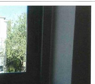
19. The window stop was missing at some windows, including at the master bedroom. The window stops are intended to prevent the windows from fully opening to prevent persons from falling out of them.
