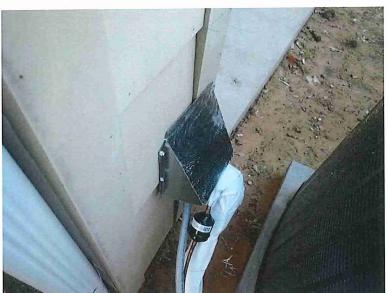
12. The air conditioning flashing hood did not extend behind the siding to the water-resistant barrier. This could leave the opening without adequate flashing that could allow water entry to the wall structure at the condensing unit.
