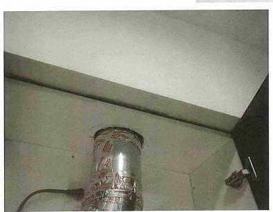
The furrdown finish was incomplete over the cabinetry at the upper cabinets at the kitchen. It appears that a valance may be missing or that the cabinets may have been installed too close to the furrdown since the cabinet doors dragged the furrdown. There may be a need to reset the cabinets lower with a valance to improve the performance and appearance.
