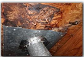
☑ Moisture stains in attic. Condition typically is caused by roof leaks; other causes or multiple causes are possible. Roof drainage problems cannot be adequately determined during dry weather. Recommend determining and eliminating source of moisture stains, and repair or replacement, as necessary.
