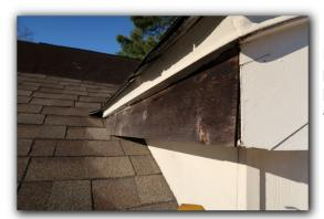
☑ Wood trim(s), eaves and overhangs (soffit). Open areas where either caulking has dried out and/or paint has started to peel could be locations of moisture penetration and related damage! Repairs are needed at this time to these areas.
