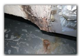
Air handler plenum/ductwork/air-conditioning unit is not properly sealed. Air is leaking from the edge seams of the blower/plenum unit in the attic. This should be sealed/taped to improve efficiency and eliminate condensation.
