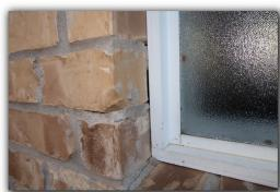
☑ Where windows meet the brick, repairs are needed.
