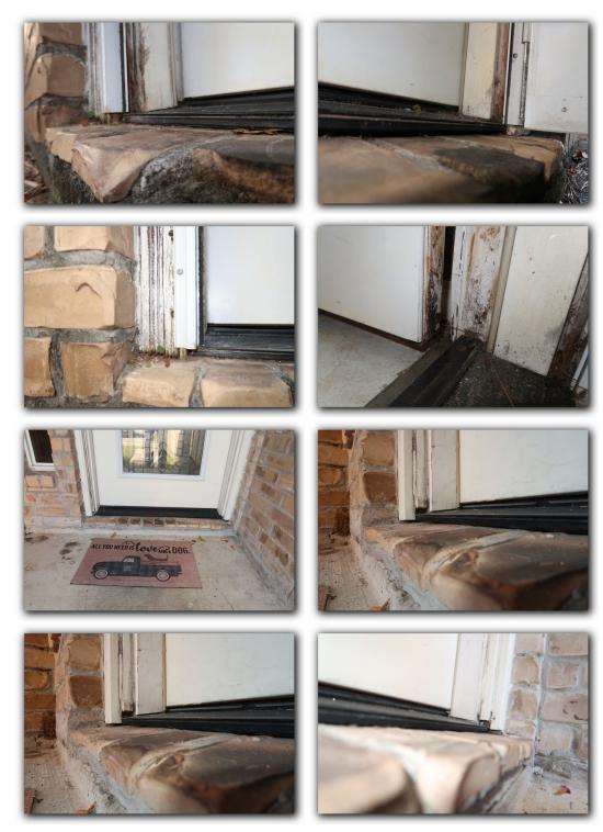
$\ \square$  The weather stripping and/or caulking around the exteriors door(s) should be improved.as well as, under the threshold should be sealed.
