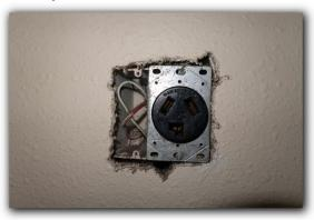
✓ Missing cover plate. Repair is necessary as this represents a safety hazard that must be corrected
