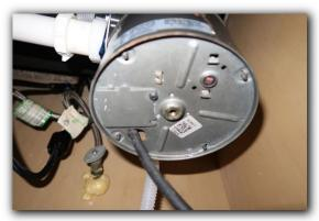
☑ Electrical wire connection is not protected from damage.
