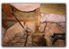
☑ Some of the insulation has been or is: improperly cut/fit, fallen out of place, missing or does not fit correctly. All of these small areas will add up to less effective insulation for the house.
