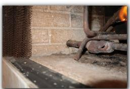
☑ The gas line entry is not sealed . A tight seal between the gas pipe and the side wall of the firebox is needed to prevent the passage of heated gases into the wall cavity. This seal should be supplied and maintained with an approved material.
