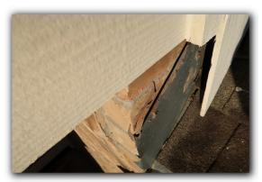
☑ Loose flashing was observed at exterior wall where the wall meets the roof. this area should be sealed to prevent water intrusion into the home
