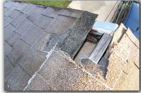
☑ Repairs to the roof system are recommended. Damaged or missing roofing material should be repaired. All roof penetrations should be examined and sealed as necessary.
