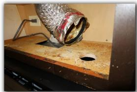
✓ Not properly connected in cabinet. Repair as necessary
