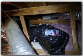
☑ The construction debris and other material should be removed from the attic or appropriately placed out-of-the-way
