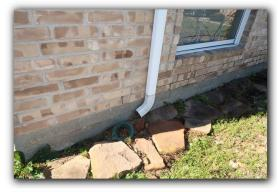
☑ At ground level, the water from the downspout should be directed at least 5 feet away from your house. It is best to have the water flowing onto a hard surface (like a driveway,a fiberglass or concrete splash guard) designed to spread the water and prohibit it puddling on the ground near your home.
