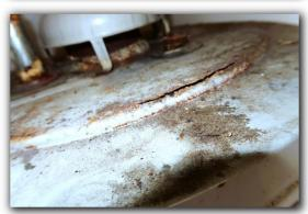
☑ Roof Leak: Type B Vent Pipe Through the Roof Deck. The water heater exhaust vent pipe was loose and/or not properly sealed, Water Leak Residue Trail was observed on the pipe at the time of inspection
