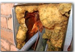
☑ Improper foam material was observed to be used to seal exterior penetrations. A none degradable/waterproof sealant is recommended in these areas.
