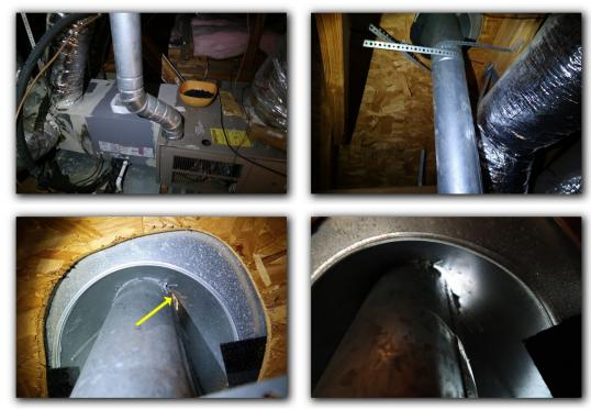
☑ Roof Leak: Type B Vent Pipe Through the Roof Deck. The furnace exhaust vent pipe was loose and/or was not properly installed, Water Leak Residue Trail was observed on the pipe at the time of inspection
