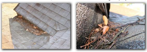
☑ Pine tree needles and any organic material on a roof especially on a valley area, then the organic material will remain wetter for an extended period of time and thus, also allow a possible growth of licen or roof algae to set root into the organic shingle causing deterioration and roof leacks. Remove the tree debri from the roof
