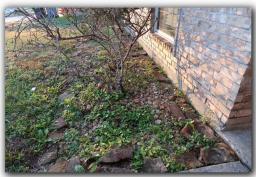
☑ Rainwater is coming off the roof and splashing up against the doors, windows, and the house. Steps (addition of gutters) should be taken to facilitate the removal of rainwater away from the foundation and eliminate the soil erosion.
