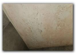
☑ There was water damage and/or black staining in the hallway bathroom celing.
