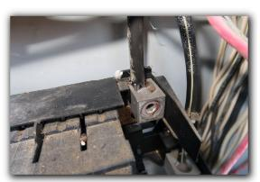
☐ The aluminum service entrance conductors were not coated with a anti-oxidant solution. This can allow the conductors to oxidized, which can be a fire hazard.
