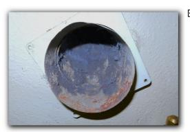
☑ The dryer's vent should be cleaned out completely before the new dryer is hooked up. This includes the termination point of the vent system. This material is very flammable. The dryer's vent should be cleaned out yearly. This material is very flammable.
