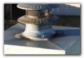
$\ \square$  Chimney cap needs to be repaired and/ or properly sealed. This is important because rain flowing down the chimney can get inside the house, attic,and/or in the firebox
