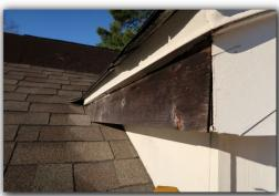
☑ Wood siding and/or fascia/trim boards has water damage in several areas. There are areas around the garage/house's siding and trim that should be repaired. It is suggested that a detailed list be compiled, prioritized and the necessary repairs started.
