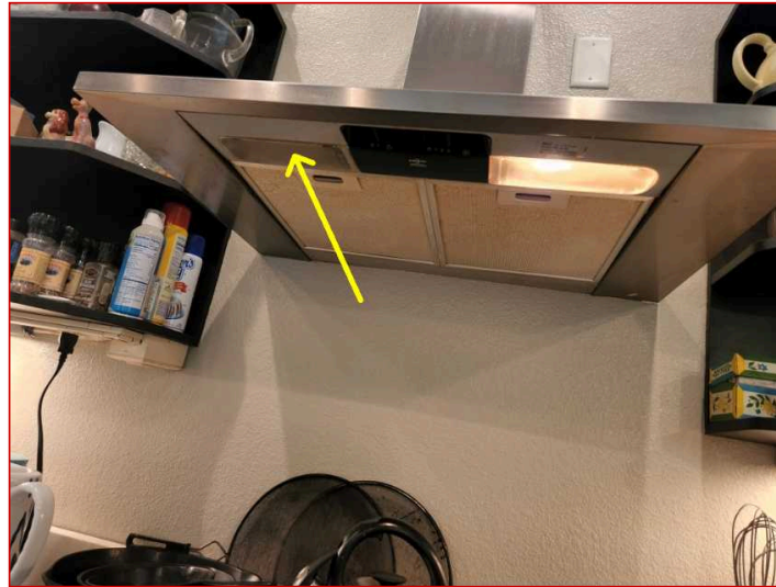
One or more of the lights not working.
