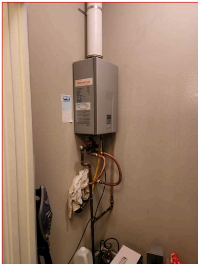
Water heater was not equipped with a corrosion resistant drain pan
