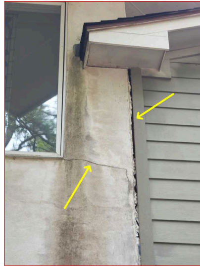
Cracks noted and should have larger trim board between walls.
