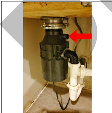
Dishwasher drain line is recommended to be tied in to the disposal
