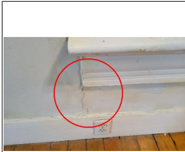
Example of cracks near windows.
