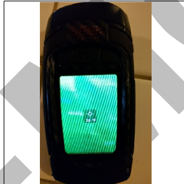
Kitchen window unit had a 36° temperature reading from the unit
