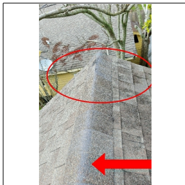
West side had minor damage or wear from the tree limbs, you can also see the granule wear
