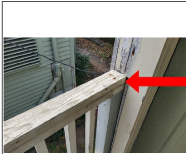
Railing is loose where it attaches to the home
