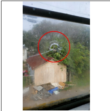
Kitchen window was damaged at the exterior of the upper pane
