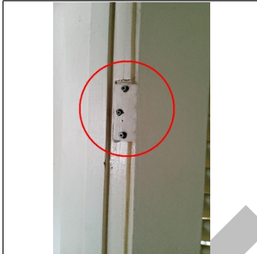
Upper hinges at door from bedroom to bathroom needs repaired
