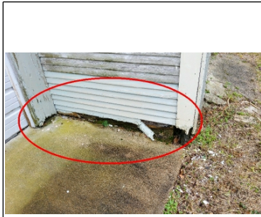
Damage to the exterior siding near garage
