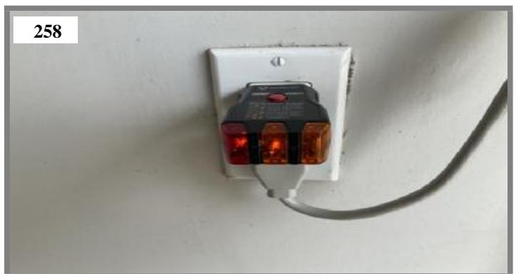
Sprinkler system outlet is hot/neutral reversed
