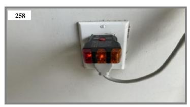
Sprinkler system outlet is hot/neutral reversed
