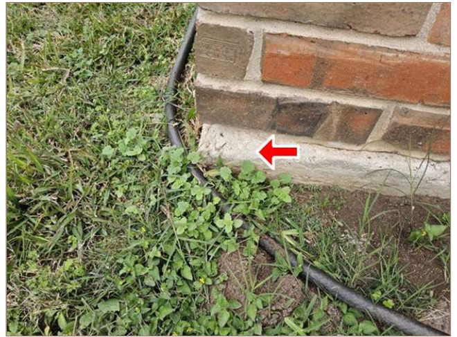
left rear corner
