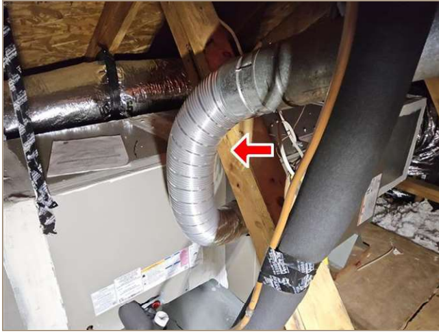
upstairs - missing B-vent
