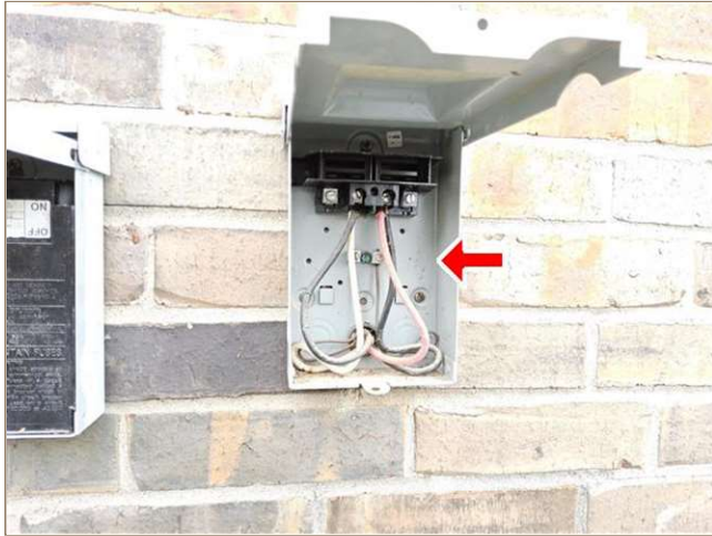
downstairs unit connected directly safety hazard
