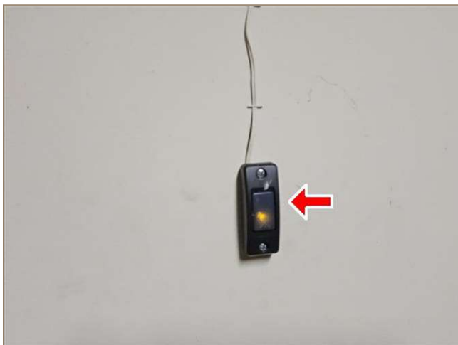
hold down switch to close
