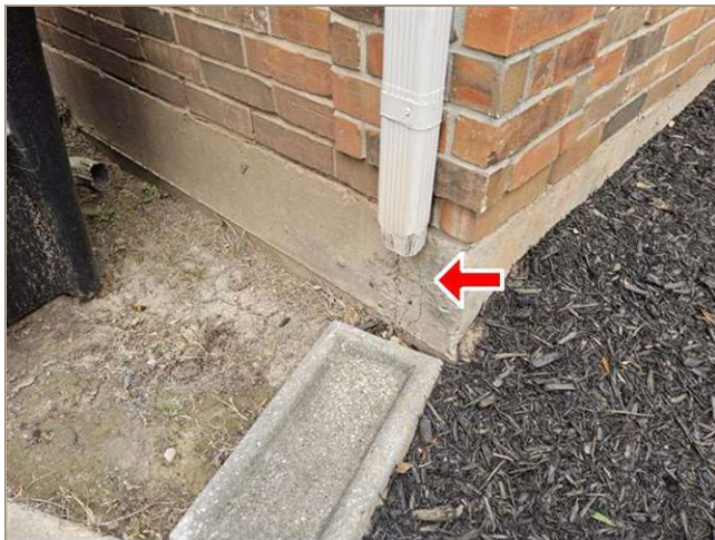
left front corner
