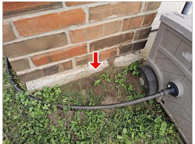
left rear corner
