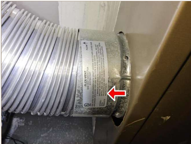
upstairs - missing B-vent
