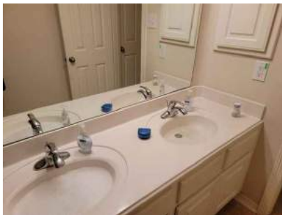
Rear Hall Bathroom Upstairs
