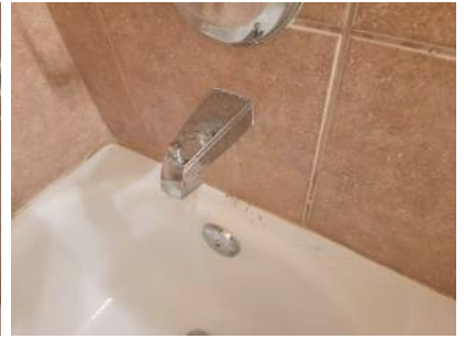
Rear Hall Bathroom Upstairs
