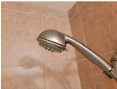
Rear Hall Bathroom Upstairs
