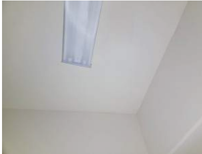
Primary Bedroom Closet
