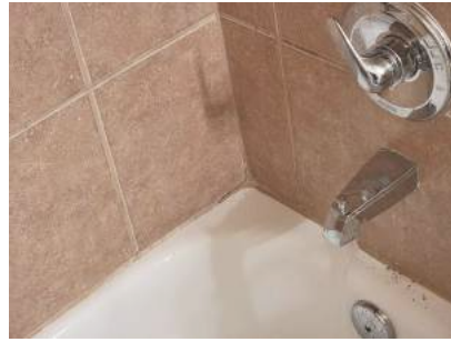
Rear Hall Bathroom Upstairs
