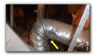
Excessive air loss at evaporator coil around drain and Freon line connections.(1st and 2nd floor unit)
