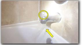
Master shower head should be cleaned or replaced as necessary, not spraying water out of the shower head ports evenly.
