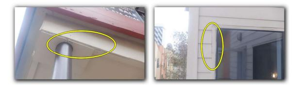
Caulking missing and/or deficient at vertical joints in siding; may allow wind driven rain entry.
