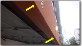
THE EXTERIOR OF THE 2328 JACSKON STREET HOME HAS BEEN CAULKED WATERPROOFED A section of small trim at the 2nd floor patio observed to be missing.
