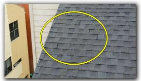
Area(s) of soft/spongy and/or rotted roof decking observed while walking on roof. (northwest, central west edge, and south center over the master bedroom)
