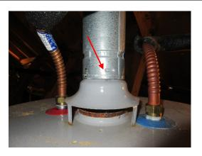
TPRV discharge pipe shall not terminate more than 6 inches above the waste receptor (ground)
