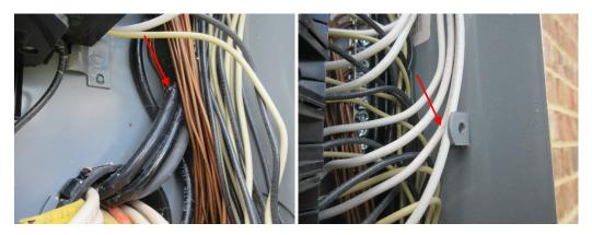
• Grounding conductors are black. Grounding conductors shall be identified by stripping the insulation from its entire length, color the exposed insulation in green, or marking the insulation in green tape at the termination.
