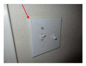
• Electrical cable shall be installed in an outlet box with a cover or receptacle installed with a faceplate
