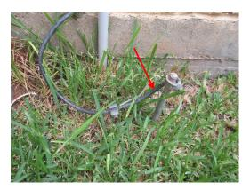
• Upper end of rod-type grounding electrodes shall be flush with or below ground level except where the attachments are protected against physical damage
