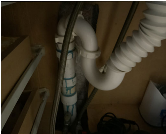
S trap and temporary drain material in place at primary bathroom
