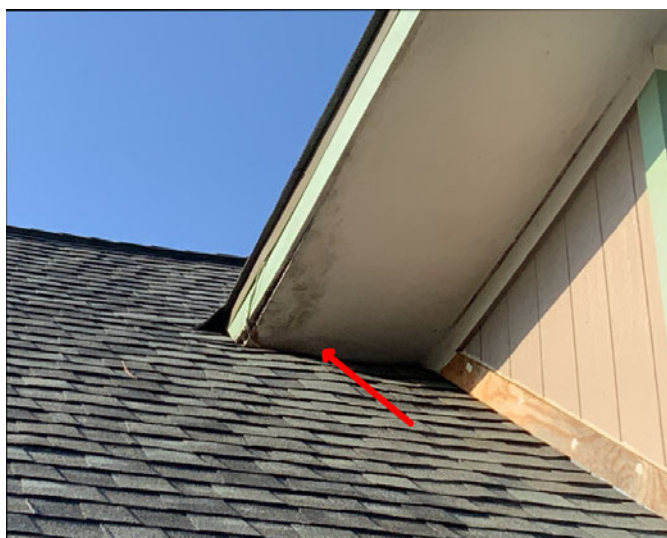
Damaged soffits
