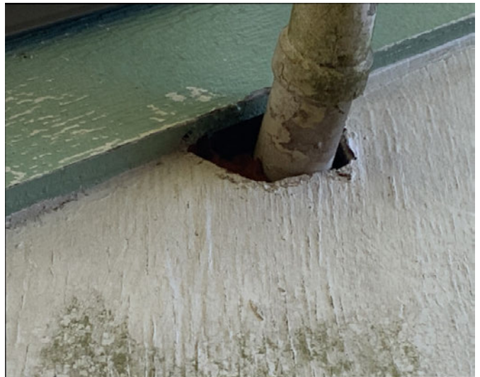
Seal all seams gaps and penetrations to home
