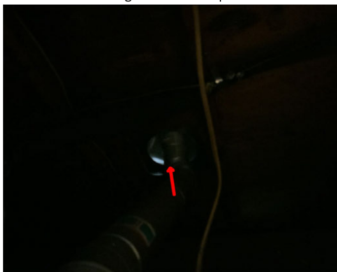
Roof jacks and flue pipes need seal improvements
