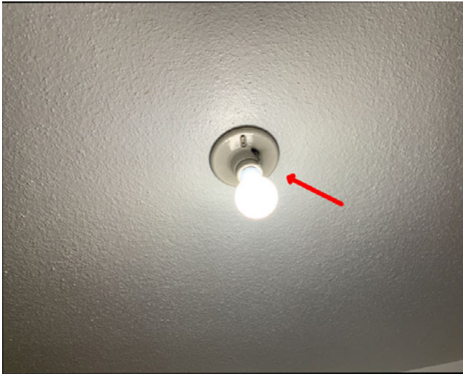
Closet bulbs are required to be protected
