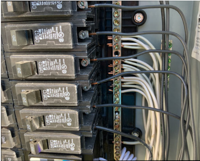
Correct all double tapping on neutral bar
