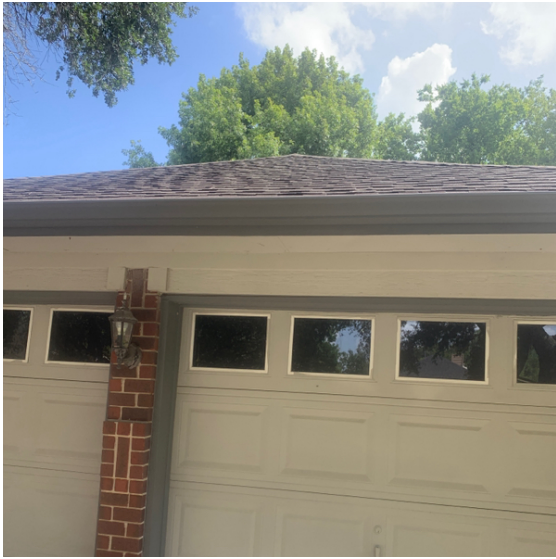
Other Treatment Photos Removed cobwebs
