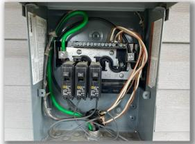
The wires entering the electrical cabinet are not properly secured or protected from the sharp edges of the cabinet.
