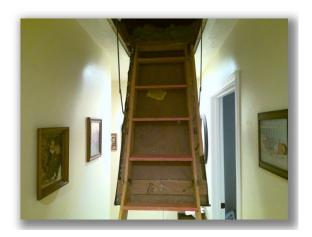
• The attic ladders in the bedroom hallway and garage are not properly installed and do not sit flush at the hinges when opened.
