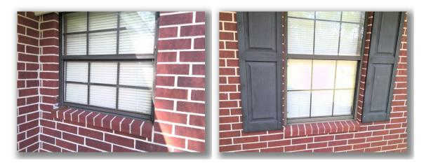
One or more of the thermal pane windows were observed to have lost their seals. This has resulted in condensation or a fog like film to develop between the panes of glass. The thermal pane windows no longer function as designed when they loose their seal and replacement may be necessary. The windows that have noticeably lost their seals are listed but may not be limited to the following: master bathroom, hall bathroom, living room, study and front corner bedroom.
