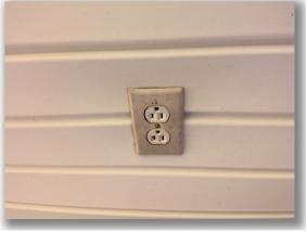
• The exterior receptacles do not appear to be connected to a ground fault circuit interrupter (GFCI)
