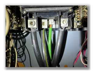
• One or more of the neutral and ground wires in the electrical cabinet were observed to be double lugged (i.e. two wires under one screw).
