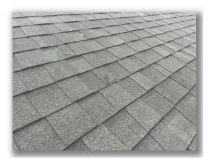
• There is excessive algae/moss growth on the roof covering on the south side of the roof covering. This can cause damage to shingles when not cleaned.
