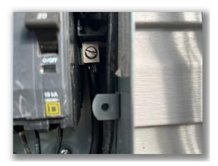
• The ground wires and the neutral wires are not properly separated in the sub-panel electrical cabinet. The neutral wires should be on their own isolated bus bar and the ground wires should be connected to the sub-panel cabinet. Although the sub-panel is functional, it does not meet current National Electrical Code standards.
