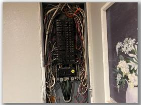
All openings (missing knockouts) in the electrical cabinet cover plate (dead front) and /or cabinet need to have fillers.
