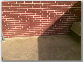
• The sidewall veneer / cladding is in contact with the roofing material. Under current building standards, there should be at least 2-inch of clearance between the roofing material and the sidewall veneer / cladding.
