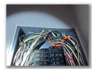
• The electrical cabinet does not appear to be properly bonded to the electrical system.
