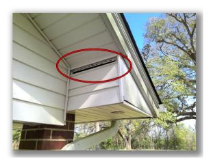
• The soffit material is sagging and/or pulling loose on the north side of the roof structure.
