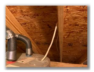
• There is no expansion tank present on the cold water supply line on top of the water heating equipment.
