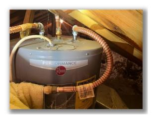
• The temperature and pressure relief (TPR) valve discharge pipe is running in an upwards direction in one or more locations. The TPR discharge pipe should run gravitationally downwards at all points.
