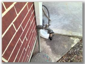
• All exposed water supply lines on the exterior should be insulated to help protect them from possible freeze damage.
