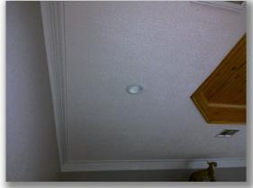
• There are not enough smoke alarms located in the home. Under current building standards, there should be a smoke alarm located in each sleeping room, outside each separate sleeping area in the
