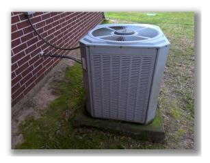
Damaged, deteriorated and/or missing insulation on the refrigerant lines should be repaired or replaced at the outside condenser.
