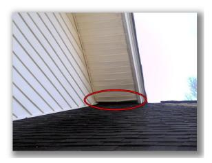
• The hatch door is not insulated at this time. This is an "As Built" condition that does not meet current energy standards. It is recommended to insulate the hatch door / opening after taking position / ownership of the property.
