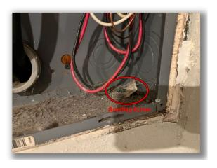
• Open electrical junction box(es) were observed in the attic area. All open junction box(es) in the attic
