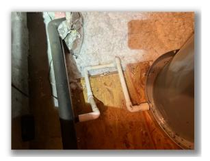
• There is no temperature and pressure relief valve (TPR) discharge pipe in place at the time of this inspection. For safety reasons, it is recommended that a TPR valve discharge pipe be installed. Under current building standards, the discharge pipe should run downward to the exterior of the structure, turn downward, and terminate within 6-inches of the ground.
