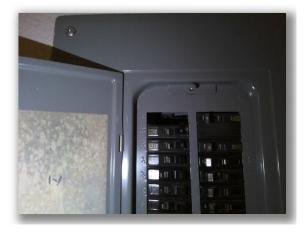
• The panel box does not have proper clearance in front of the cabinet. The panel box cover plate (Dead
